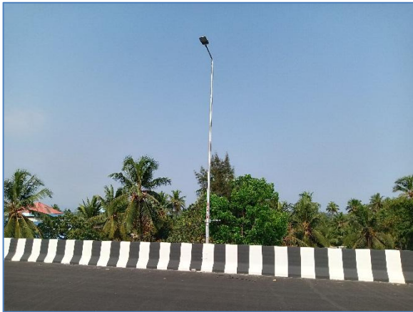
Segmental Lighting @ Km 231.155 Median
