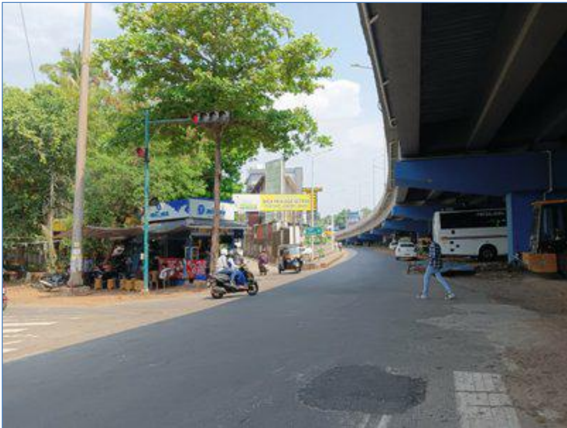
A View of Project Corridor with 5m wide Slip Road @ Km 245.700 LHS
