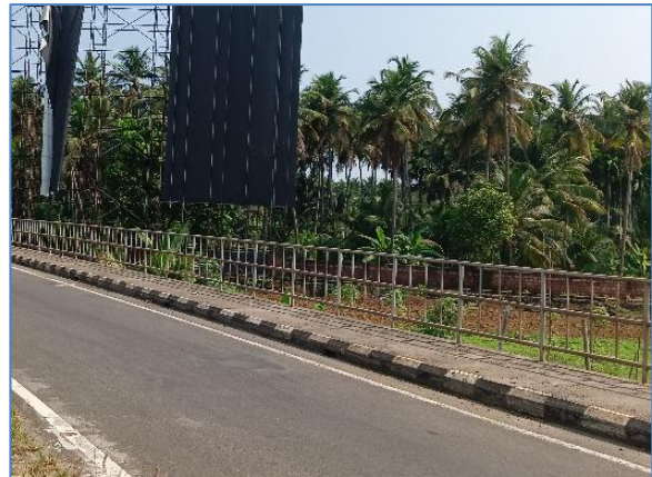
RCC drain cum Footpath at km. 258+793 RHS
