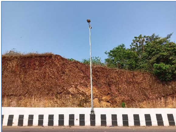
Single Arm lighting on Service Road @ Km 234.551 RHS
