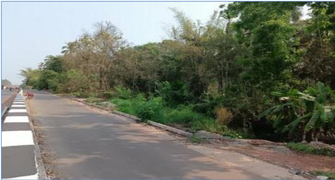
A view of the Project Corridor with 5.5m wide Slip Road at Km 242.060 RHS
