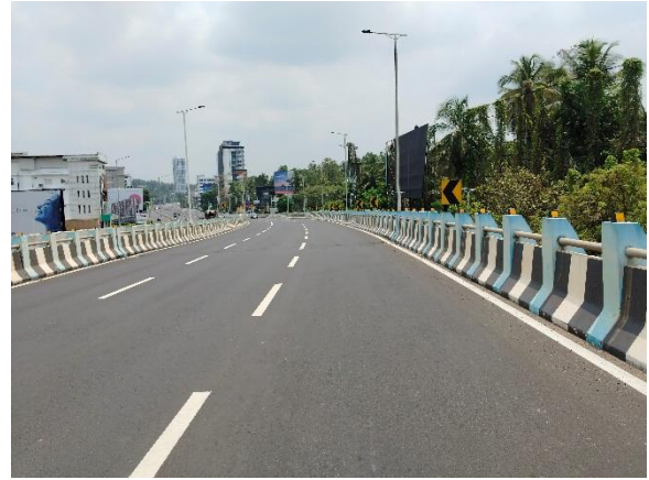
Single Arm lighting @ Km 246.600 RHS
