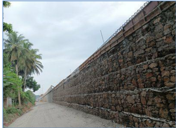
Gabion Wall at km. 254.500 - RHS
