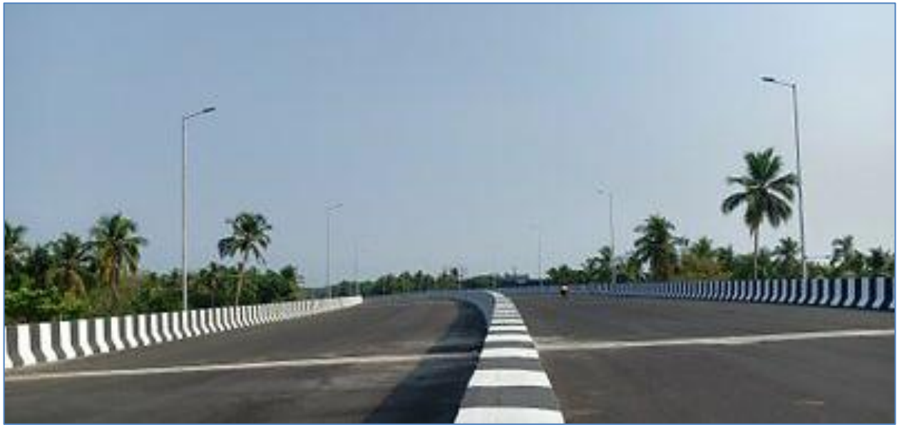
View of the Project corridor at Km. 231+400 with a 6-lane configuration in the main carriageway (MCW) with Segmental Arm Lights on Shoulders and provided with CCB on Median.
