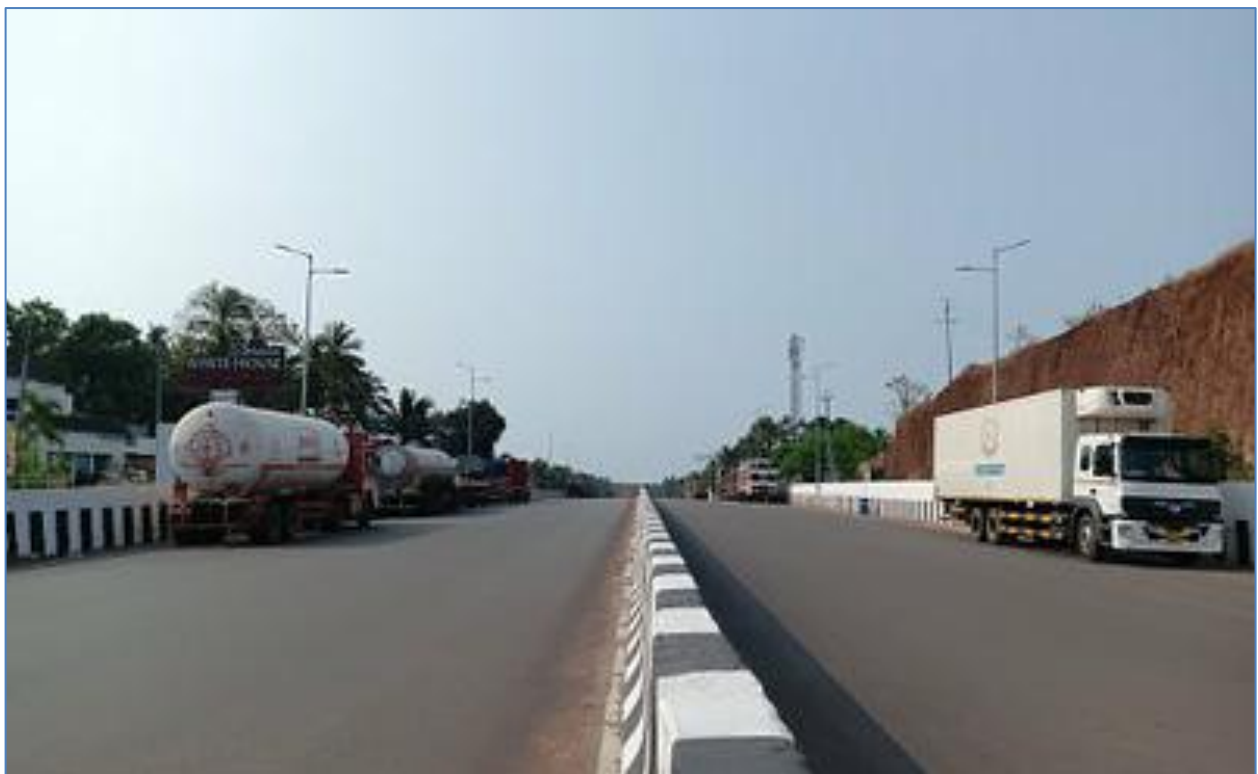
View of the Project corridor at Km. 234.600 with a 6-lane configuration in the main carriageway (MCW) with CCB on median
