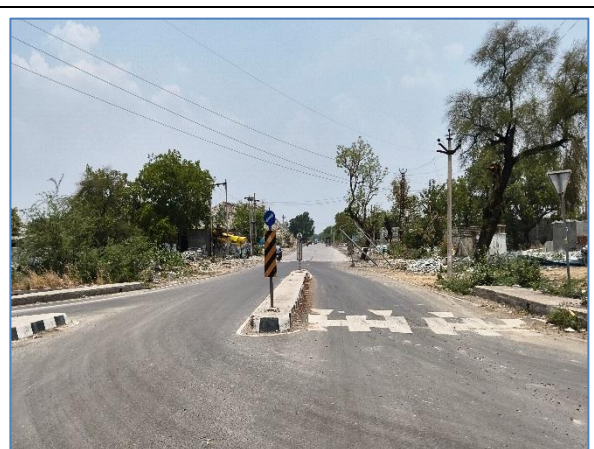
Major Junction at km 27.000 BHS
