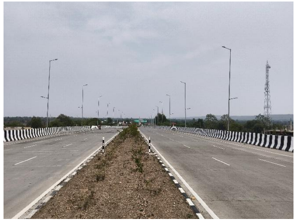
A view of double arm Lighting BHS at km 58.000
