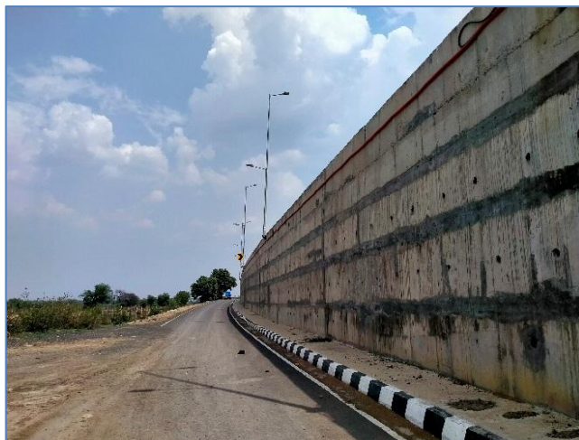
RCC Wall at km-32+600 RHS
