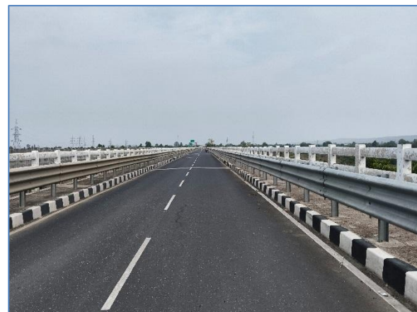
A view of the Project Road at km 57.000 RHS
