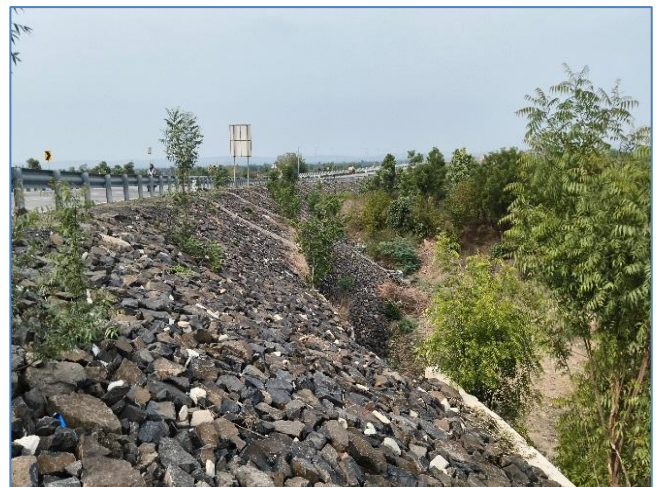
Stone Pitching at km-56+900 RHS
