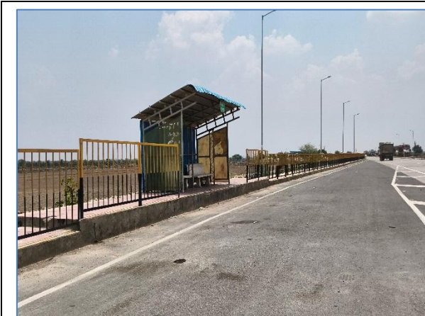
Bus Bay with Bus shelter @ Km 13.550 RHS
