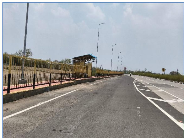
Bus Bay with Bus shelter @ 22.000 LHS
