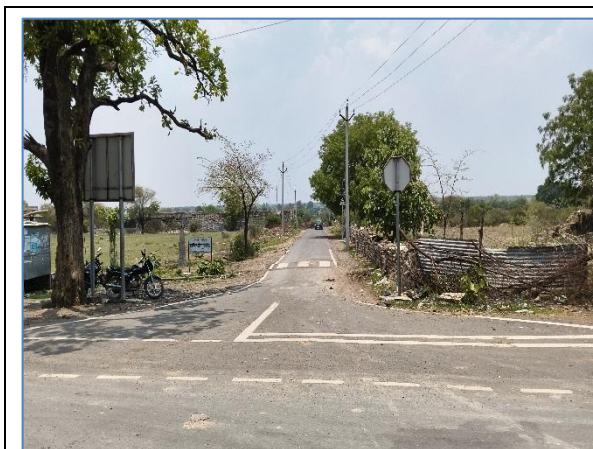
Minor Junction at km 19.900 BHS
