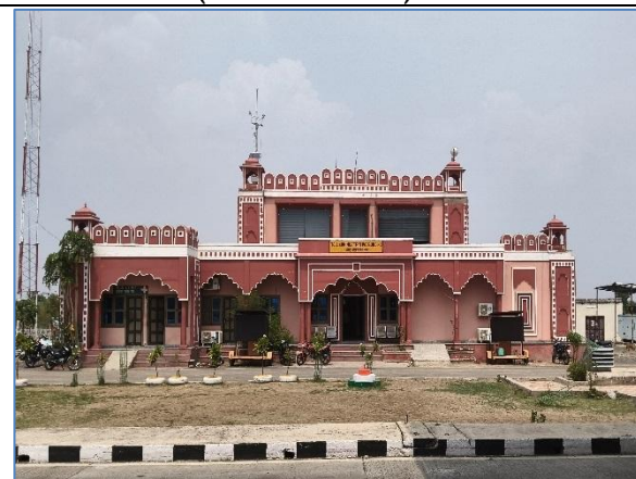
Toll Admin Building @ km 27.700
