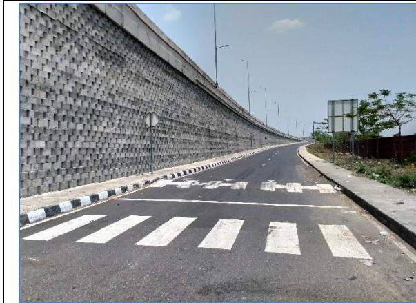
Service road at km 50.100 LHS
