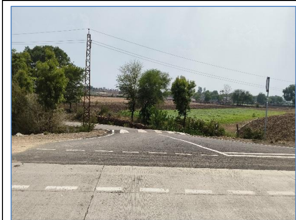
Minor Junction at km 32.550 BHS
