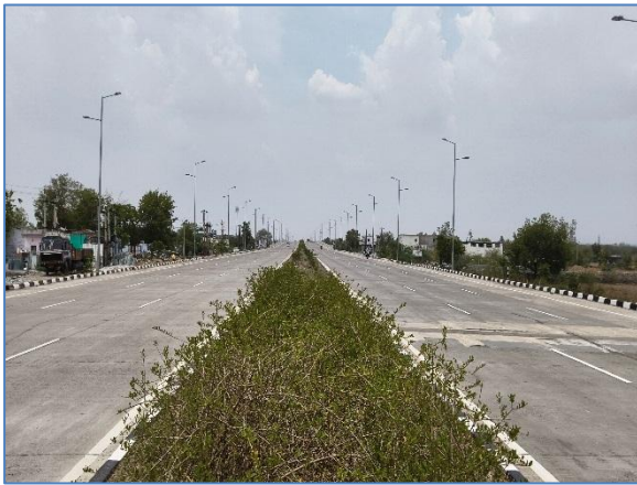
A view of the Project Corridor at Km 32.000
