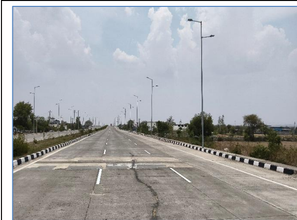
A view of Double Arm lighting at km 42.000
