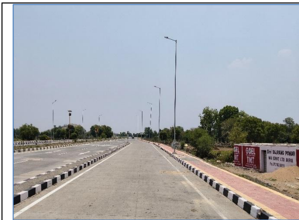
A view of Single Arm lighting at km 18.200 RHS
