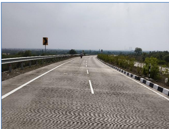
A view of the Project Road at km 52.000 LHS
