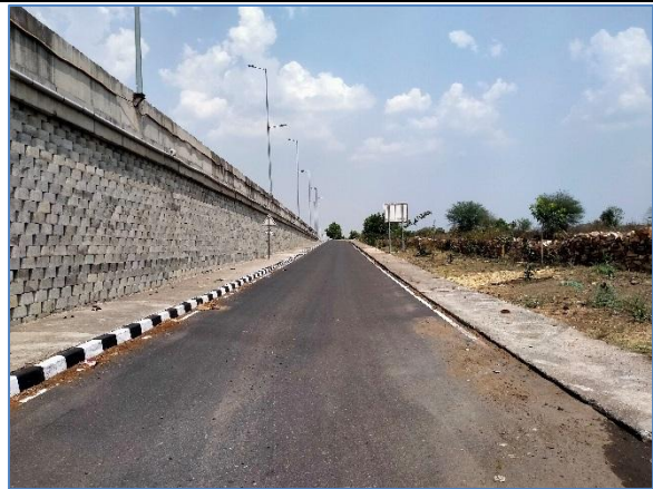
Service road at km 38.500 RHS
