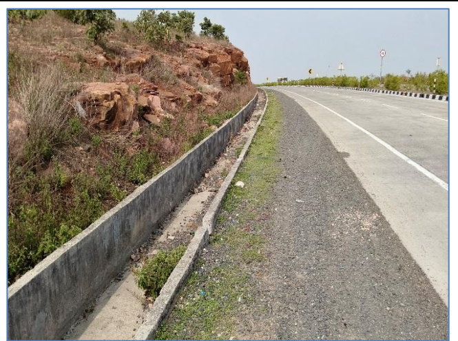
RCC Open Lined Drain at Km 52+300 LHS
