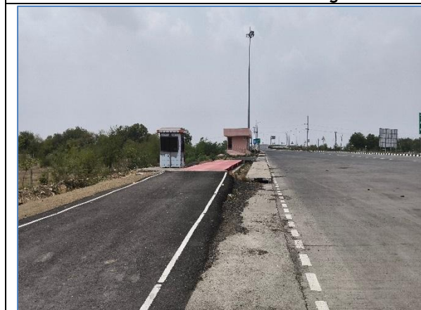
Static Weigh Bridge @ km 27.700
