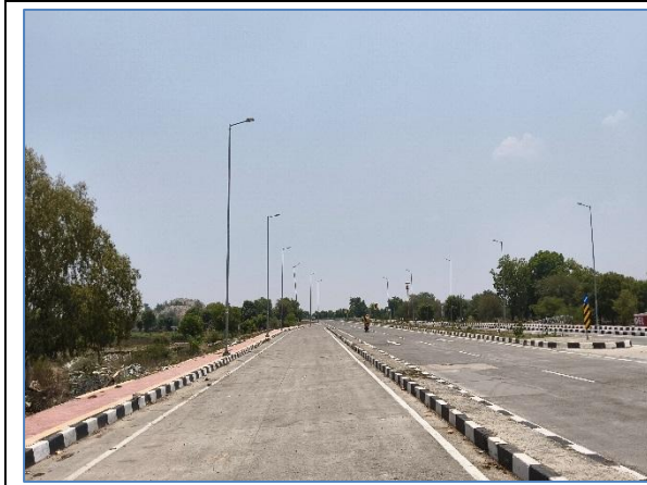
A view of Truck Lay Bye at Km 18.100 LHS
