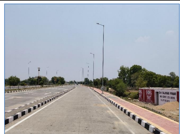
A view of Truck Lay Bye at Km 18.100 RHS
