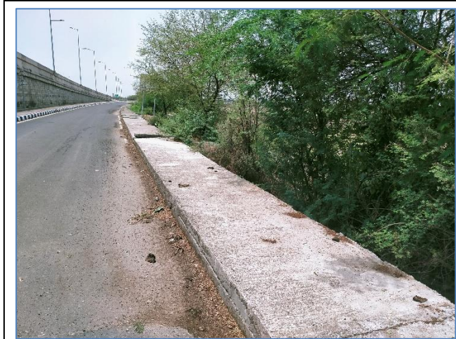
RCC Cover Drain at Km 12+550 LHS
