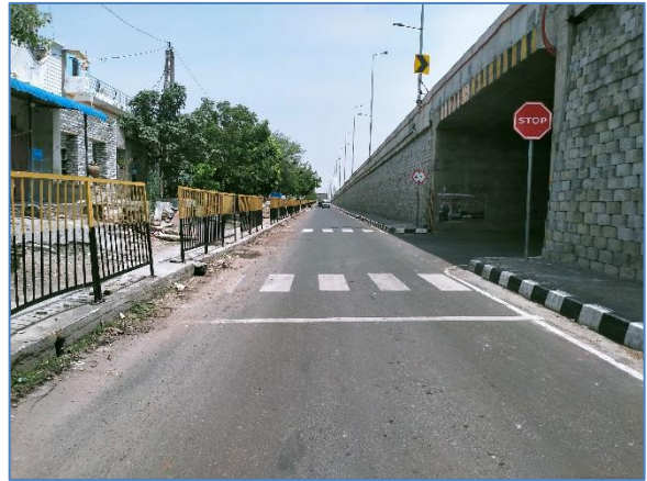
A view of the Project Road at km 24.600
