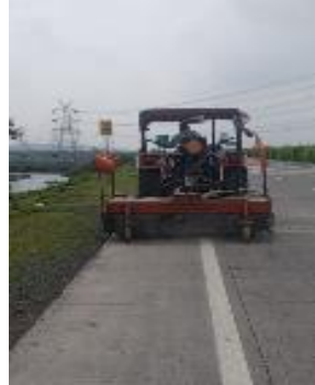
Mechanical road cleaning
