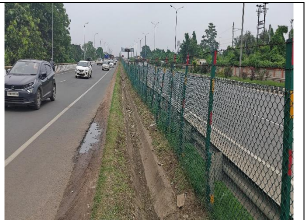
Drain at Km 655+300 LHS
