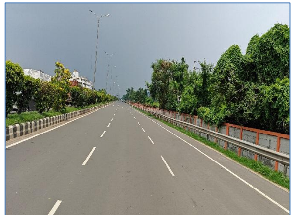
A view of the Project Road at km 654.900 RHS
