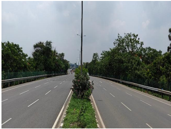
A view of the Project Road at km 653.400
