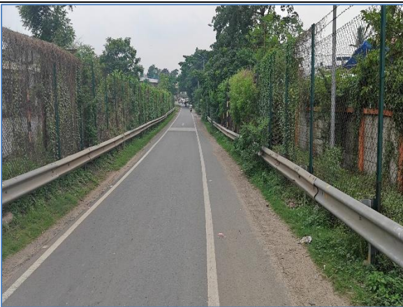
View of Ramp-E
