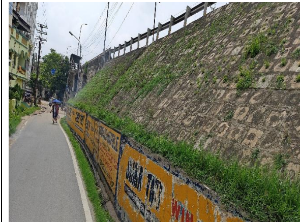
Partial RCC wall Km 655+160 LHS
