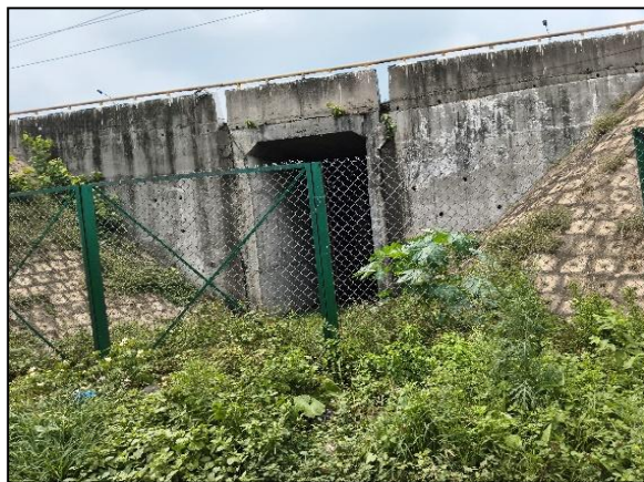
Box Culvert at 655+052
