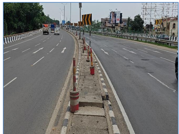
A view of the Project Road at km 656.000
