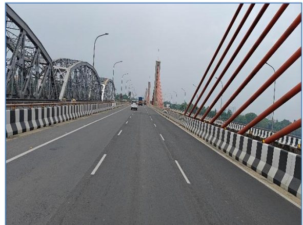
A view of the Project Road at km 657.000
