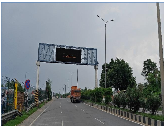
A view of the Project Road at km 655.560
