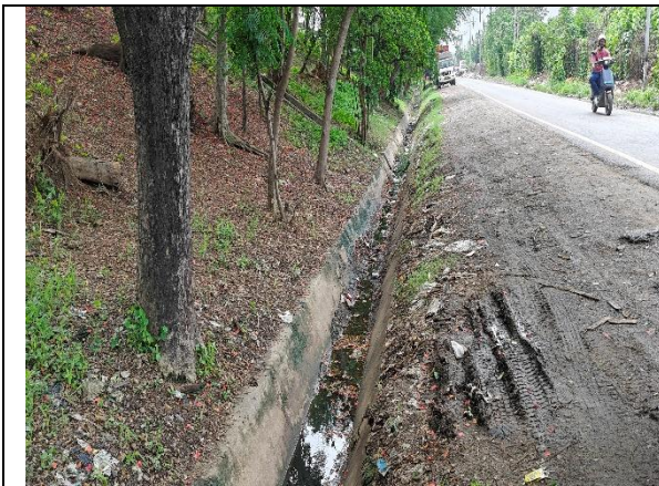
Drain at Km 653+500 RHS
