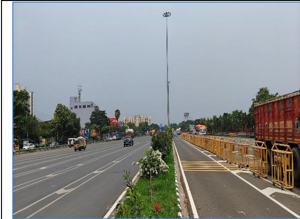
High Mast Lighting at km 654.100 on MCW
