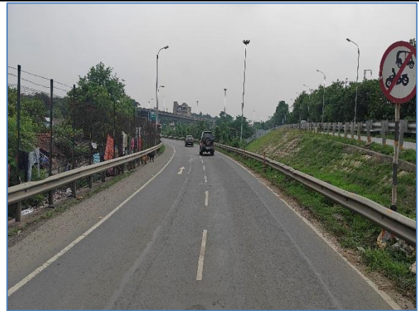
High Mast Lighting at km 658.000 Ramp-B
