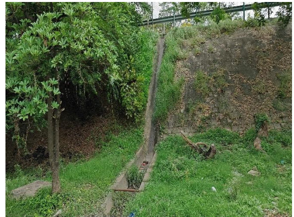
High Embk. with chutes km 653+600 RHS
