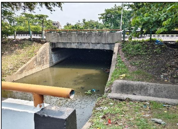
Box Culvert at 653+607
