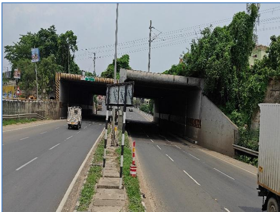
A view of the Project Road at km 656.100
