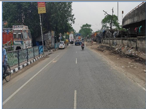
View of PWD-Down road
