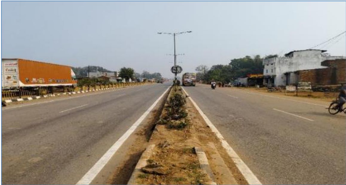
A view of the Project Corridor with 9.5m wide carriageway on both sides of 1m wide Median at Km 158.000
