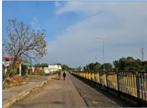
5.5m Wide service road @ Km 182.500 LHS
