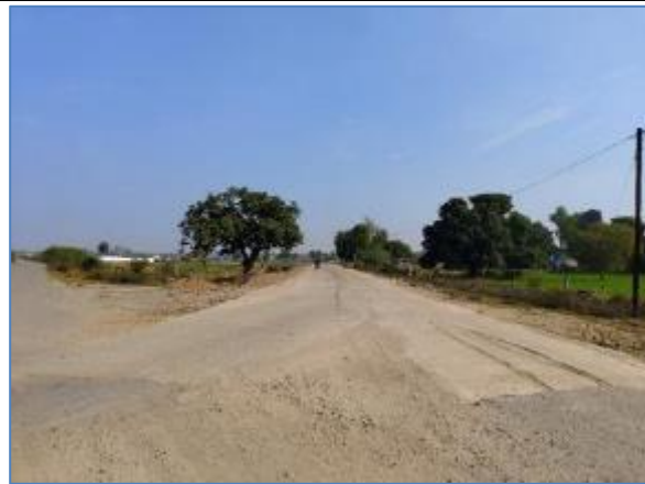
Minor Junction @ Km 222.490 LHS
