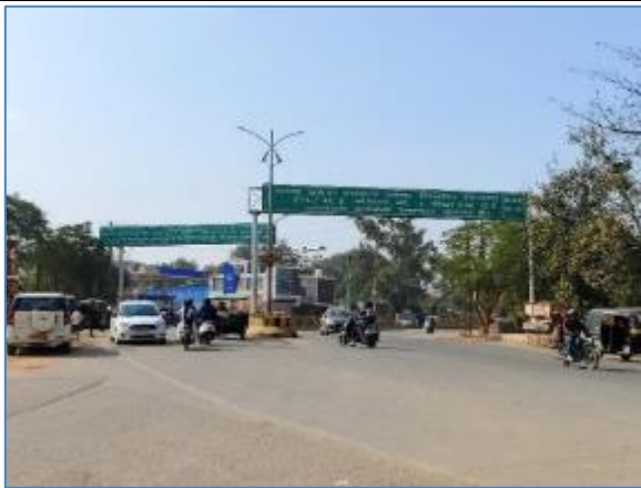
Major Junction @ Km 229.850 LHS
