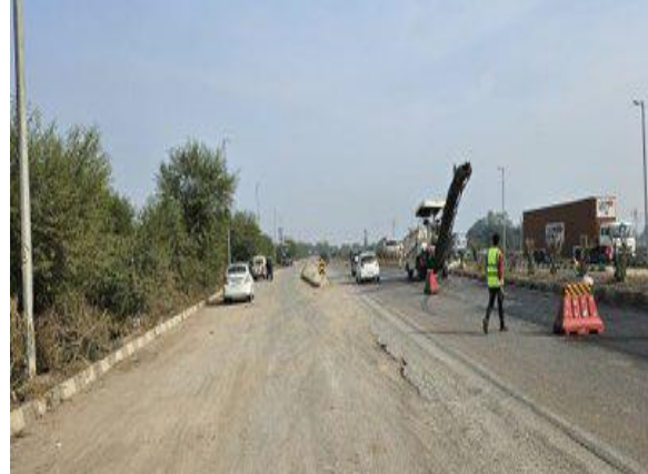
Truck lay-bye @ km 221.700 RHS
