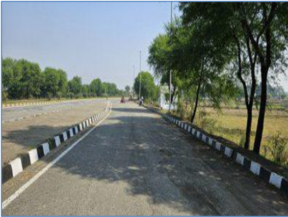
Truck lay-bye @ km173.400 LHS
