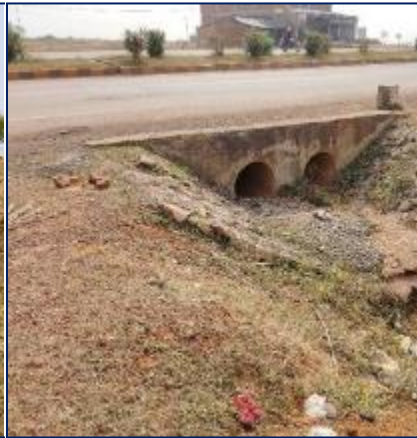
Pipe Culvert at Km 153+785
