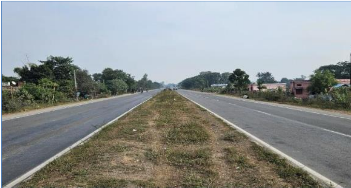
A View of Project Corridor with 4.5m wide Median @ Km 214.200
