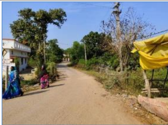
Minor Junction @ km 227.140 RHS
