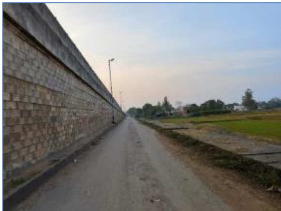
Single Arm lighting on Service Road @ Km 161.000 RHS
