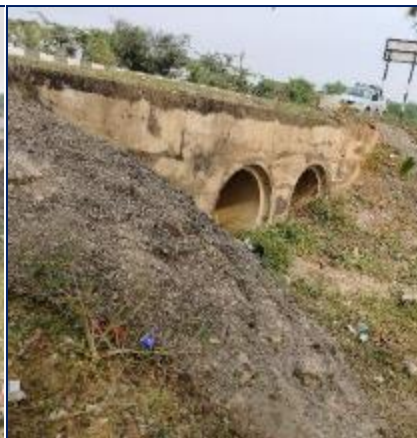
Pipe Culvert at Km 153+785
