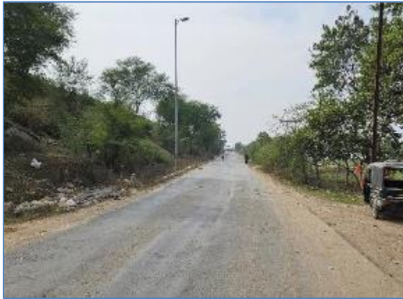
7m wide Service Road at Km 205.700 RHS
