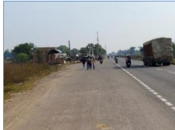
Bus-bay with shelter @ km 218.920 RHS
