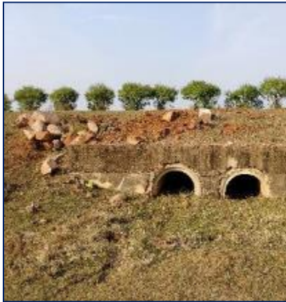
Pipe Culvert at Km 143+150
