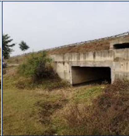
Box Culvert at Km 172+380
