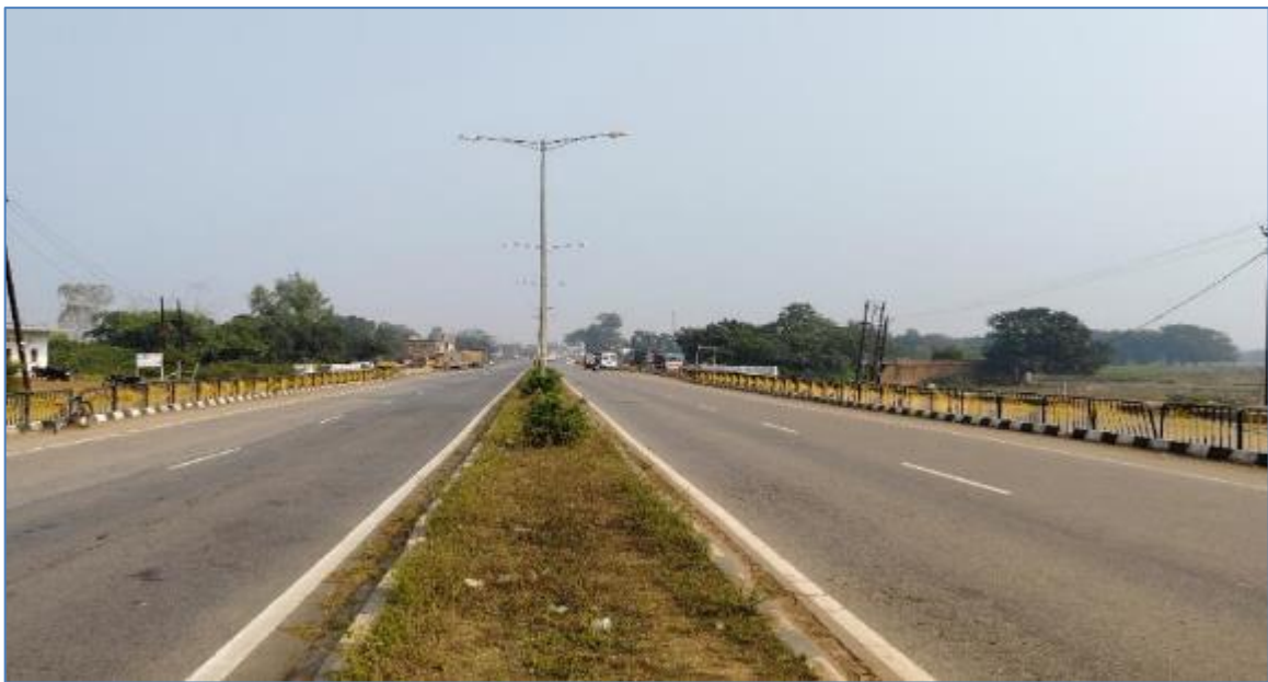
A view of the Project Corridor with Double arm lighting in the 2 m wide Median & PGR on separators on BHS at Km 159.000
