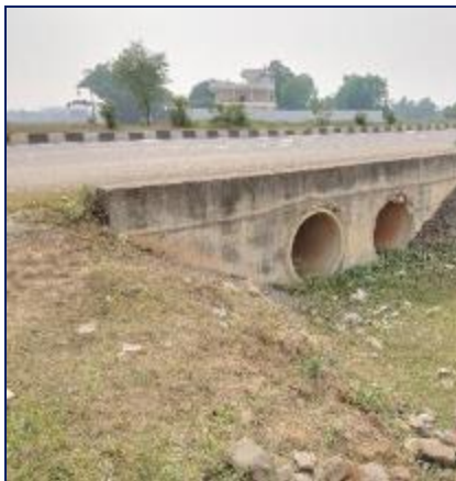
Pipe Culvert at Km 143+150
