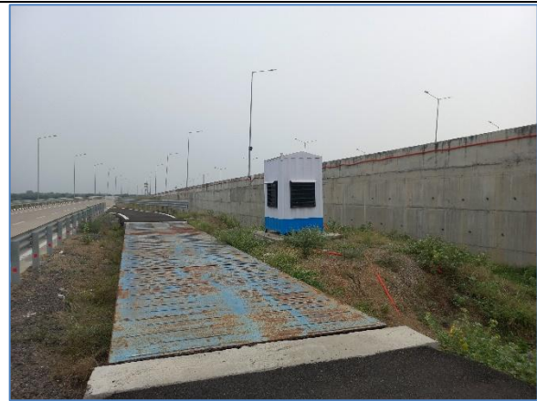
Static weigh Bridge at Km322.800 @ RHS Ramp
