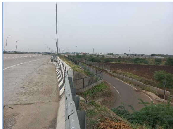
Connecting Road at km 318.980 RHS
