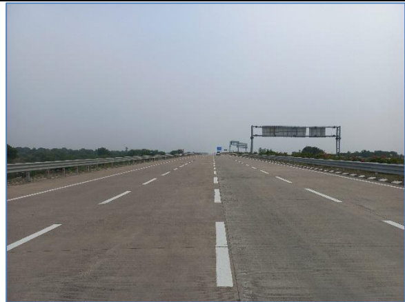
Fair Condition @ Km 322.000 RHS
