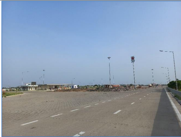
Rest Area at km 306.500 LHS
