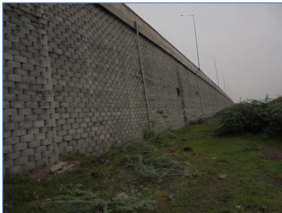
RE Blocks at km 299.350 LHS
