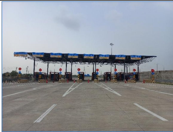
Exit Toll Plaza at Km322.800 @ LHS Ramp
