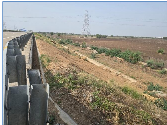
RE Blocks at km 299.350 LHS
