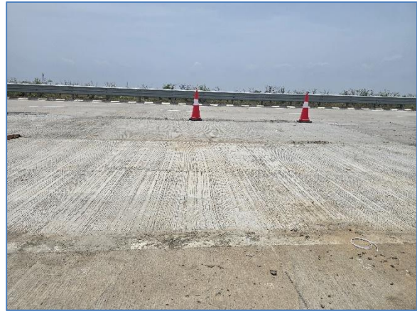
Panel Repair works Done @ Km 310.800 RHS
