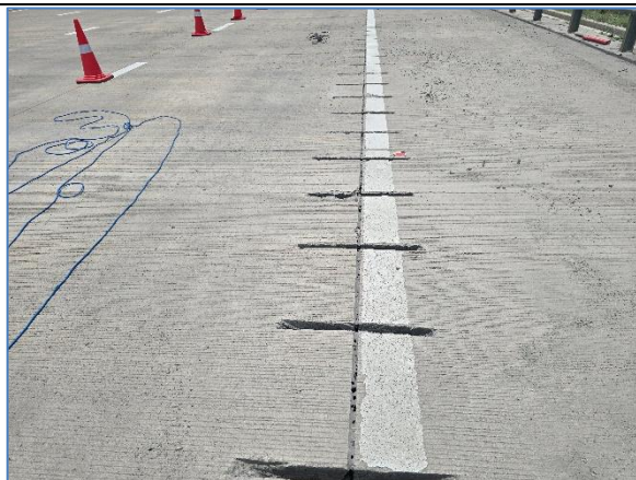
Longitudinal Wide Joint Repair work in progress @ km 310.480 RHS
