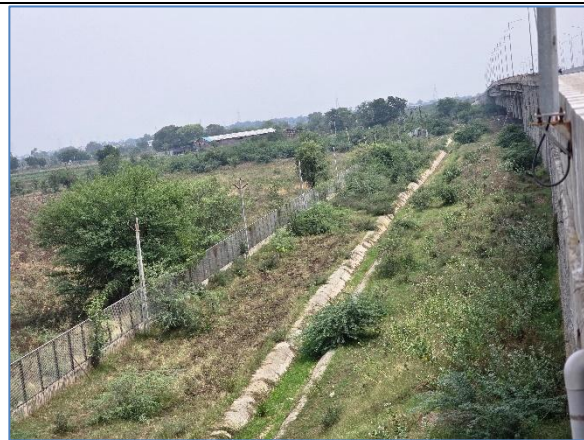
Trapezoidal Drain at km 292.600 LHS
