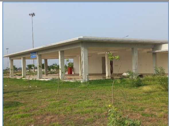
Dhaba at km 306.500 LHS Rest Area
