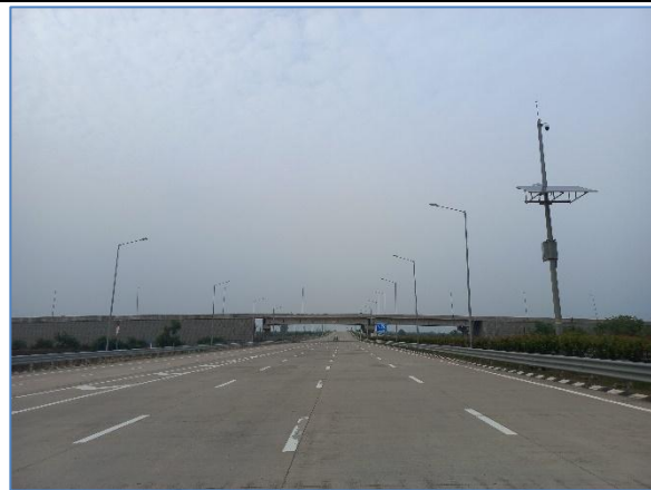
A view of the Project Road at km 306.000
