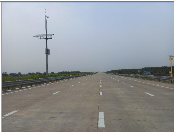
A view of the Project Road at km 316.000
