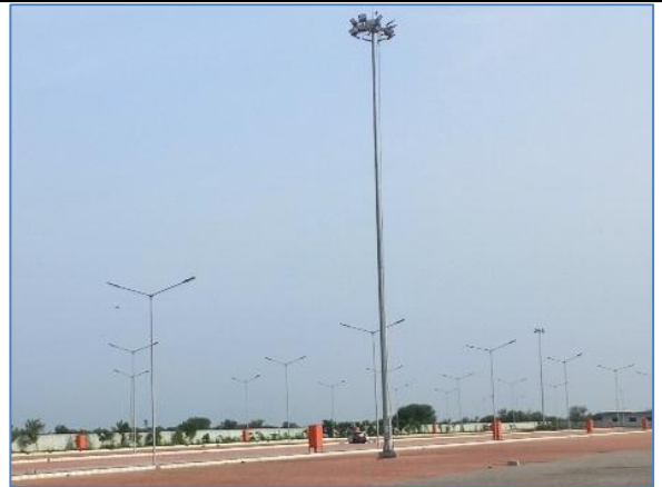
High mast at km 306.530 LHS
