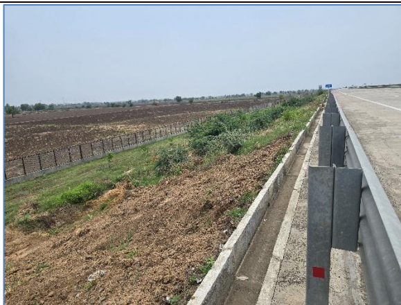
Lined Drain at km 302.900 LHS
