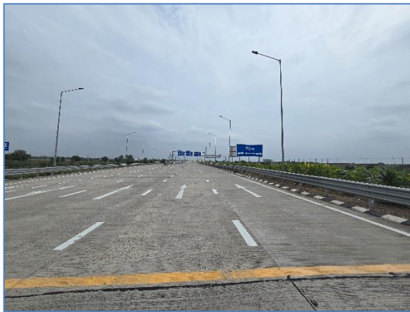
A view of the Project Corridor at Km 292.000
