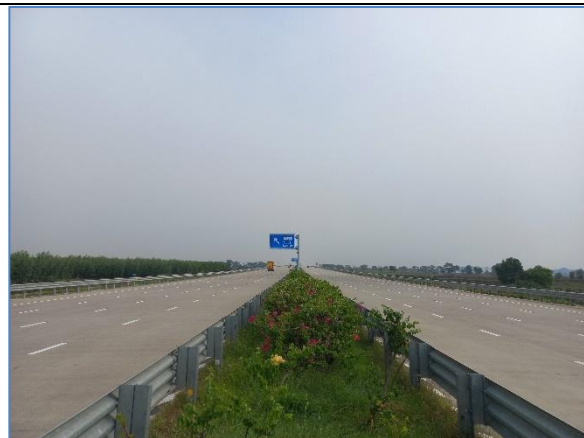
A view of the Project Road at km 320.000
