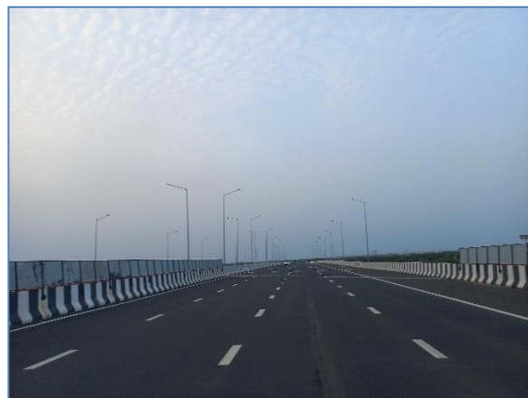
A view of the Project Road at km293.000
