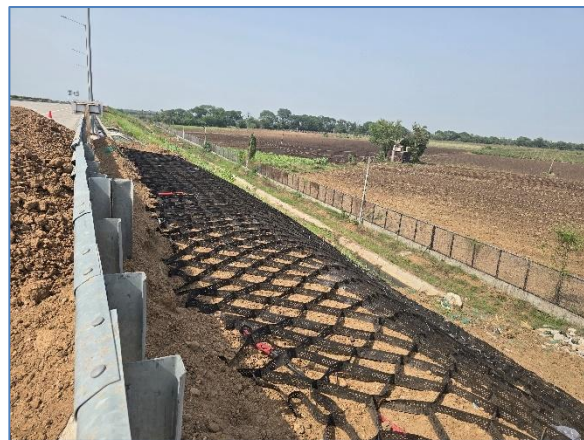
Repair works of Embankment at km 318.440 RHS
