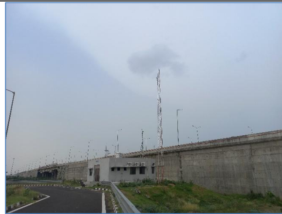
Admin Building at Km322.800 @ LHS Ramp
