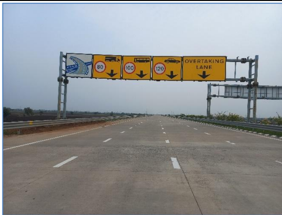
A view of the Project Road at km 302.000
