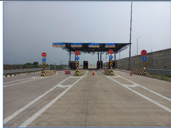
Entry Toll Plaza at Km322.800 @ RHS Ramp
