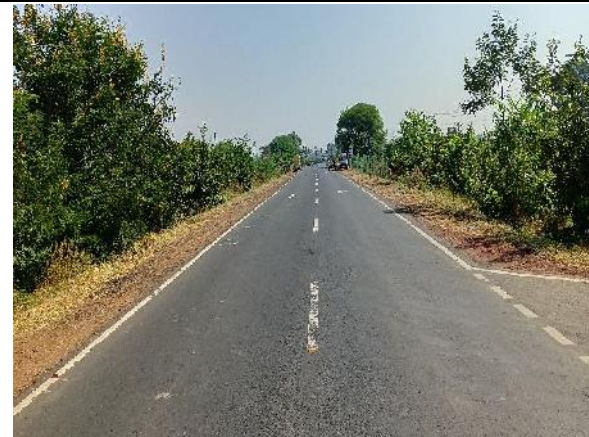
A view of Project Road Km: 218.000
