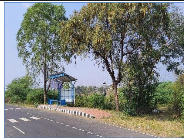
Bus Bay & Bus shelter @ Km 51.450 - LHS_SH - 294
