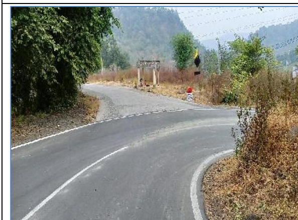
Minor Junction at km 8+200 - LHS_MDR - 66
