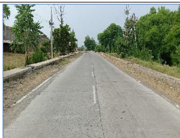
A view of Project Road (SH-305) Km:53.100
