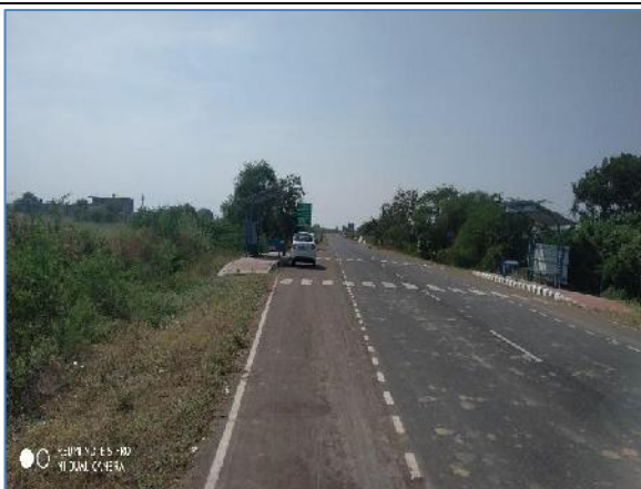
Bus bay with shelter @ Km 71.750-BHS
