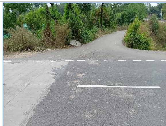
Minor Junction at (SH-305) km 47.150 -RHS
