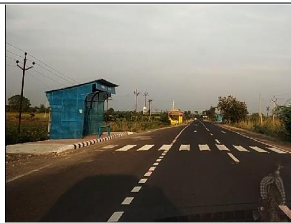
Bus bay @ Km 195.200-LHS
