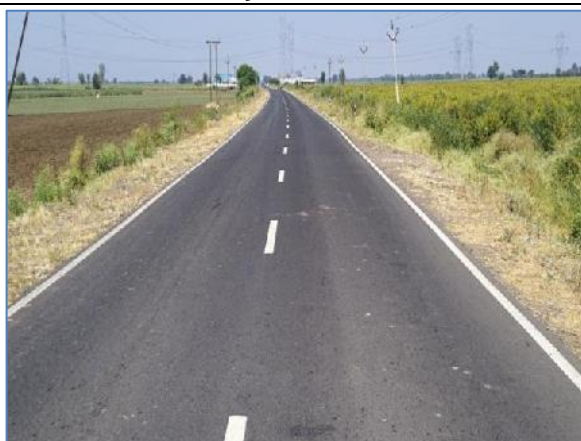
A view of Project Road Km: 34.000
