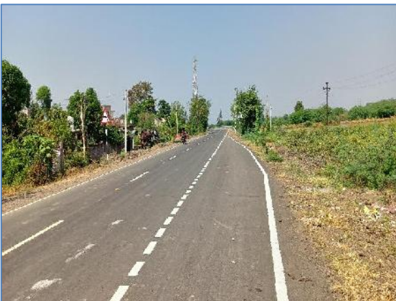
Bus bay @ Km 14.000
