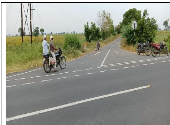
Minor Junction at km 196.00-LHS
