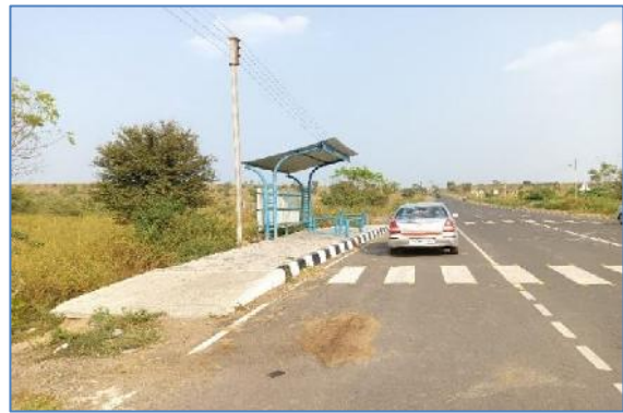
Bus bay with shelter @ Km 28.875 -SH-296
