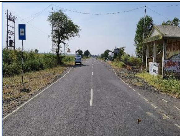
A view of Project Road Km: 69.145, Package 6
