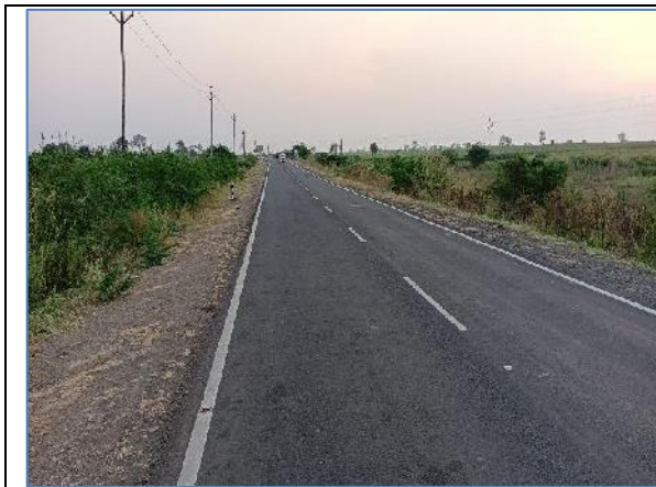
A view of Project Road with 7.0m wide at Km: 4.000_SH-312, Package-1
