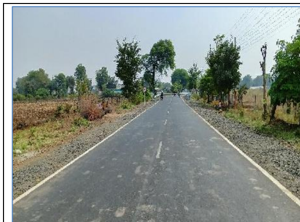
A view of Project Road (SH-305) Km: 56.000
