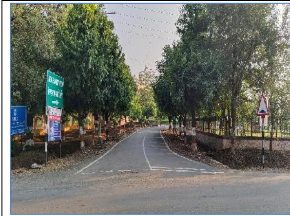
Minor Junction at km 95.450 - RHS_SH - 280
