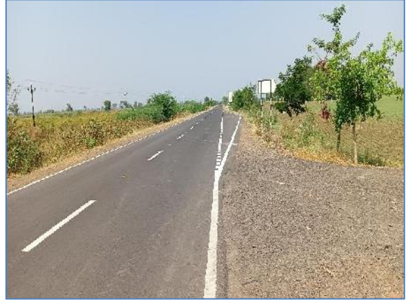
Bus bay @ Km 17.500
