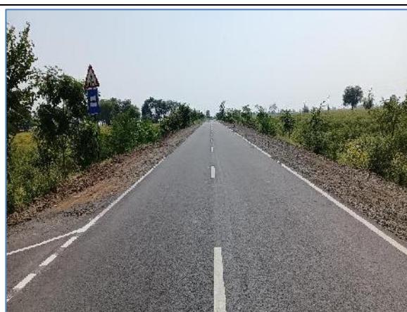
A view of Project Road Km: 18.000
