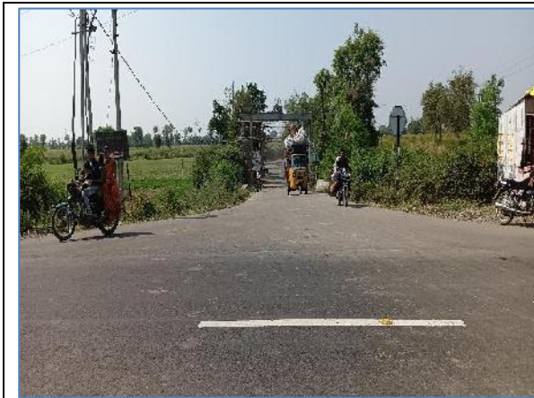
Minor Junction at km 8+680 - LHS
