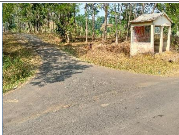
Minor Junction at (MDR-8) km 8.200 -LHS
