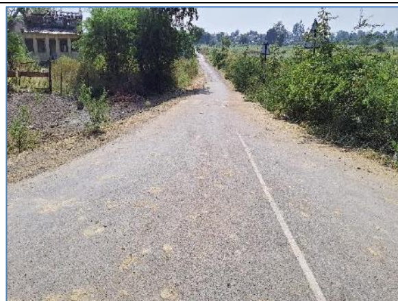
Minor Junction at km 66.567-LHS
