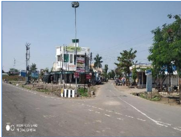
Minor Junction at km km 78.970 -RHS
