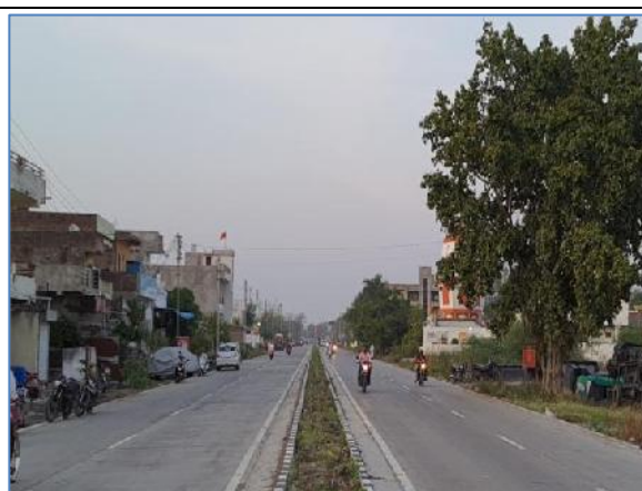
A view of Project Road Km: 28.000
