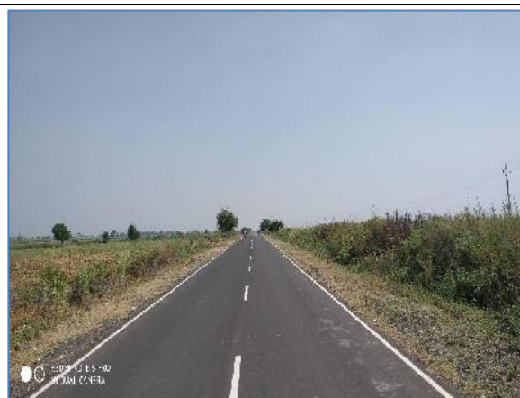
A view of Project Road Km: 79.000
