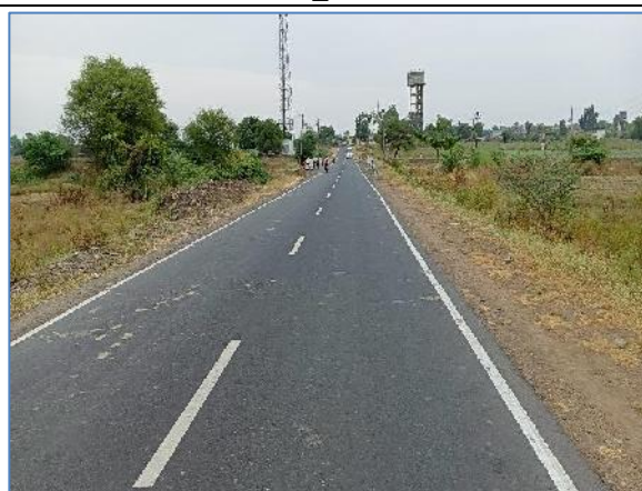
A view of the Project Road with 7.0m wide With at Km: 13.000_SH-280
