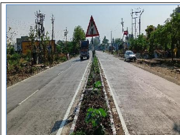
A view of Project Road Km: 1.000
