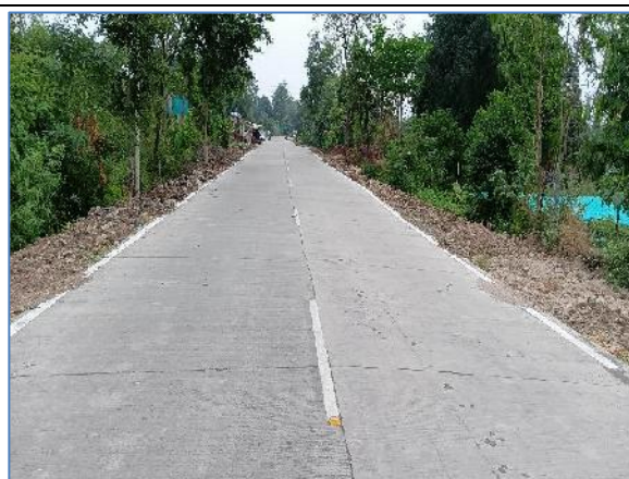
A view of Project Road (SH-305) Km: 47.200
