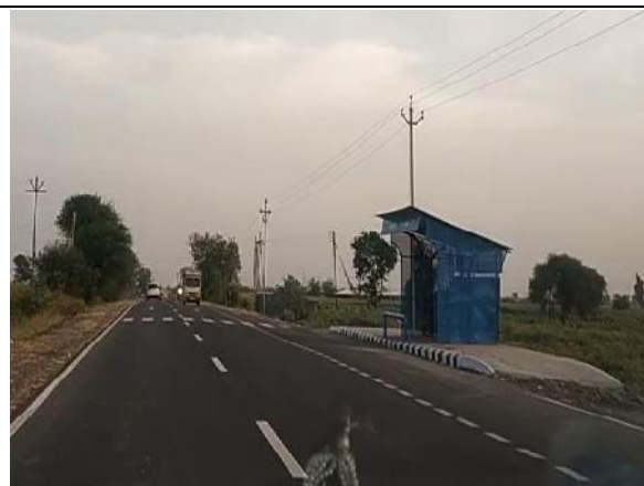
Bus bay with Bus shelter @ Km 201.050-RHS
