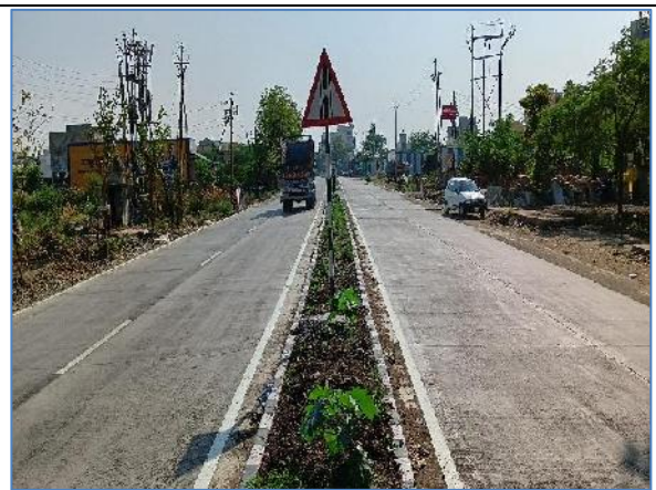
A view of Project Road Km: 1.000 -Package 2
