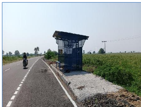
Bus Bay with Bus shelter @ Km 23.200
