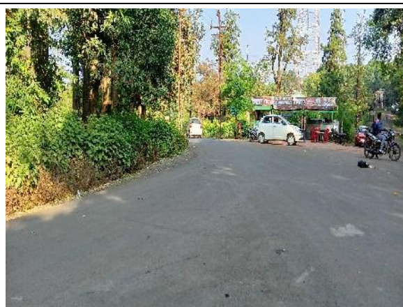
Major Junction at (SH-305) km 24+000 -BHS
