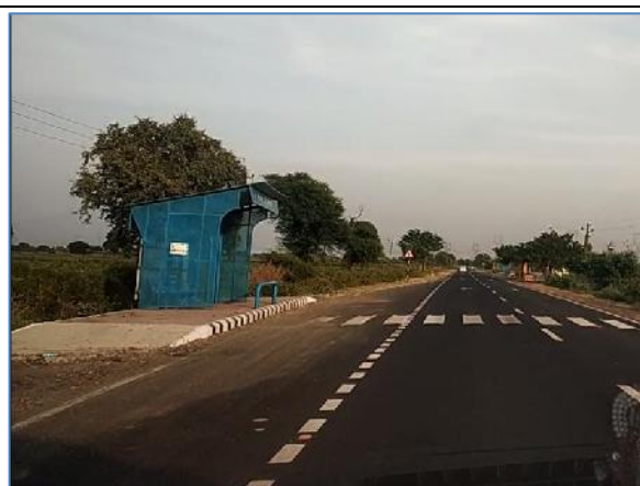
Bus bay with Bus shelter @ Km 193.720-LHS
