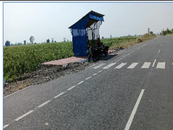
Bus shelter @ Km 6.200-LHS_SH-312
