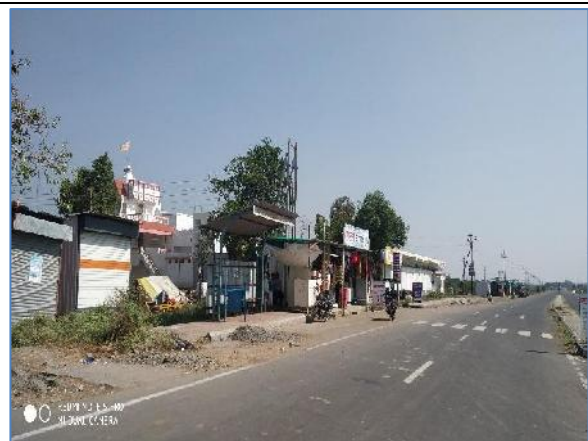
Bus Bay with Bus shelter @ Km 85.620-LHS
