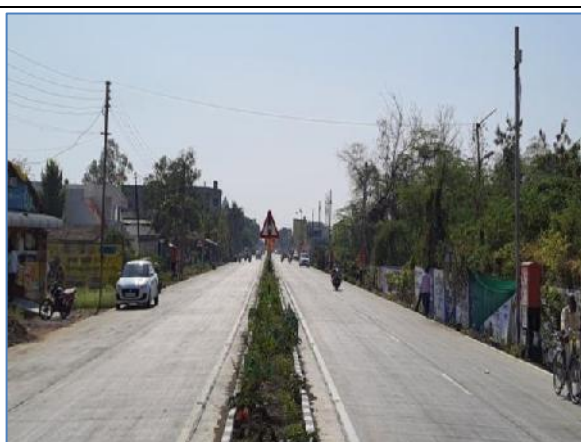
A view of Project Road Km: 27.885
