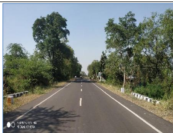
A view of Project Road Km: 88.150
