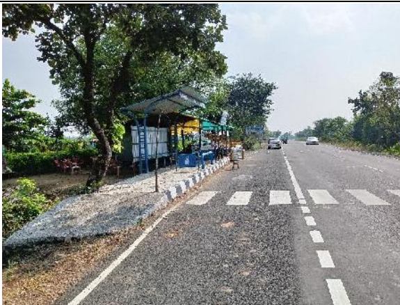
Bus Bay with Bus shelter @ Km 23.850 -SH-297
