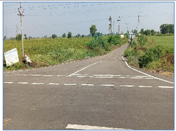
Minor Junction at km 14+060 - LHS
