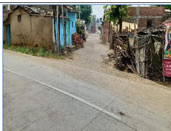
Minor Junction at km 15+250 - LHS_MDR - 66
