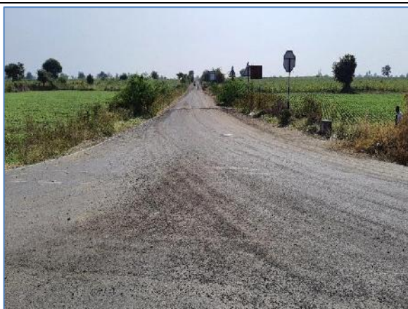
Major Junction at km 65.250 -RHS
