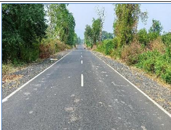
A view of Project Road (SH-305) Km: 50.000
