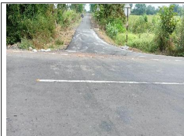
Minor Junction at km 21+400 - LHS_MDR - 45
