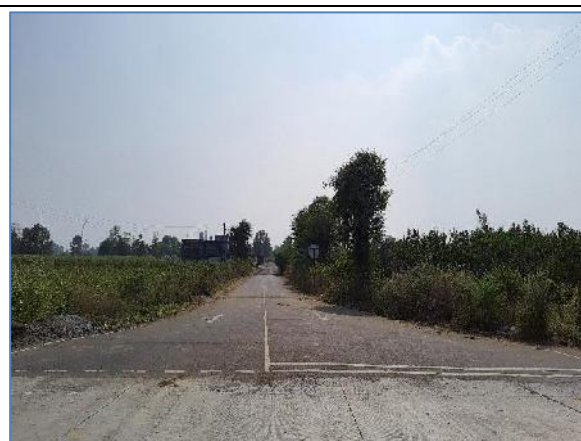
Major Junction at km 46.400 - RHS_SH - 294
