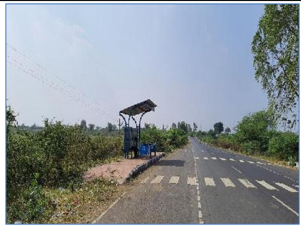
Bus Bay & Bus shelter @ Km 51.450 - LHS_SH - 294
