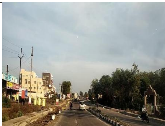
A view of Project Road Km: 181.100, Package 4
