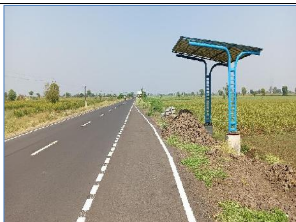
Bus Bay with Bus Shelter @ Km 19.350 (Bus Shulter Under Construction)
