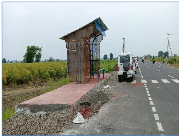
Bus Bay with Bus shelter @ Km 20.700-RHS_SH-280
