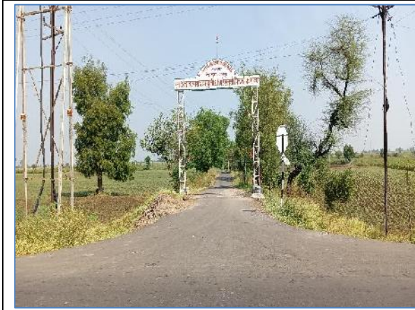
Minor Junction at km 11+820 - LHS
