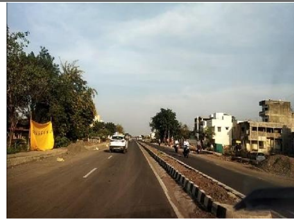
A view of Project Road Km: 182.800
