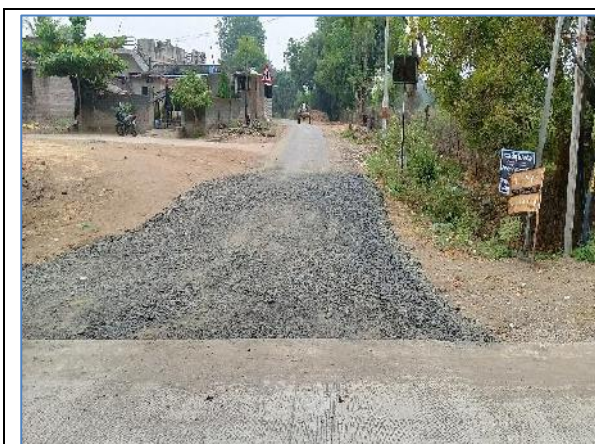
Minor Junction at km 14+900 - LHS_MDR - 66
