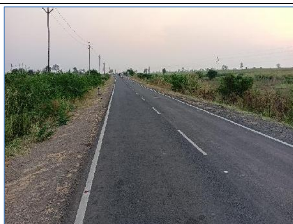
A view of Project Road with 7.0m wide at Km: 4.000_SH-312
