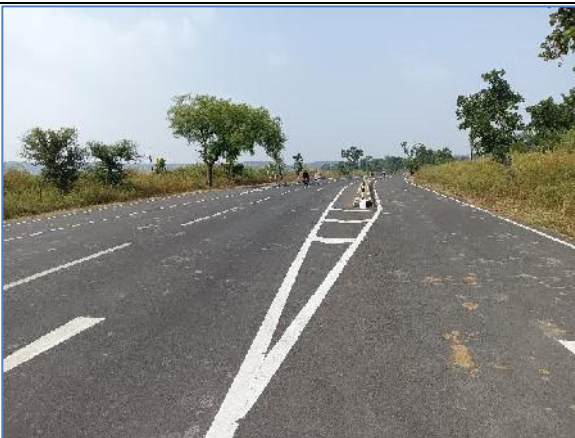
Truck lay bye@ Km 14.400 -SH-297-RHS
