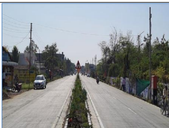
A view of Project Road Km: 27.885, Package-3
