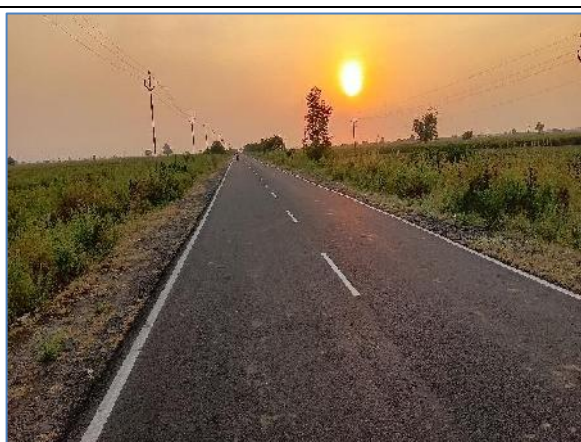
A view of Project Road with 7.0m wide at Km: 1.000_SH-312
