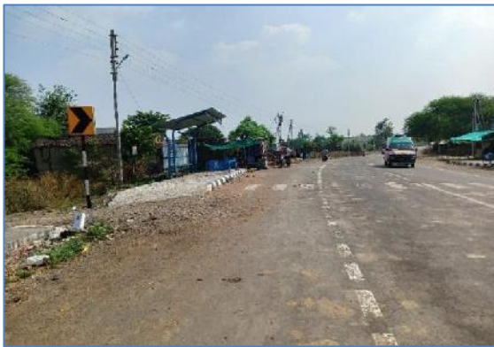
Bus bay with Bus shelter @ Km 19.650-SH-297
