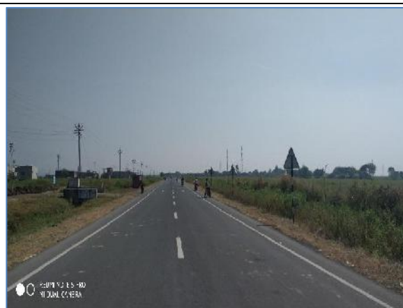
A view of Project Road Km: 86.000
