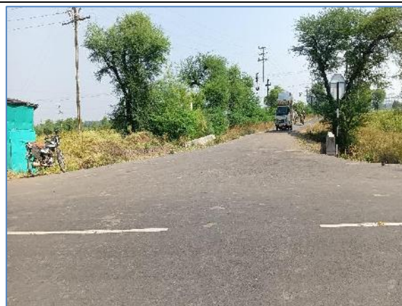
Minor Junction at km 6+040 - LHS
