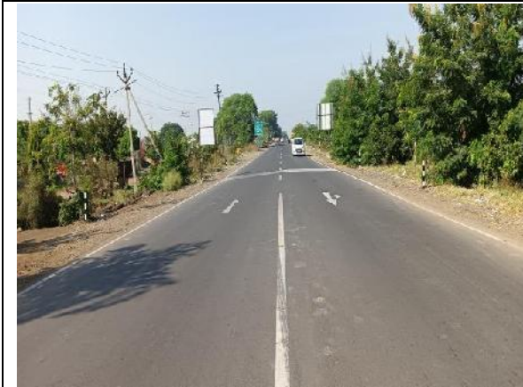
A view of Project Road Km: 224.000
