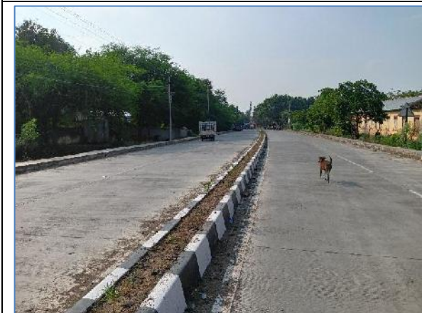
A view of Project Road Km: 26.500 -SH-296
