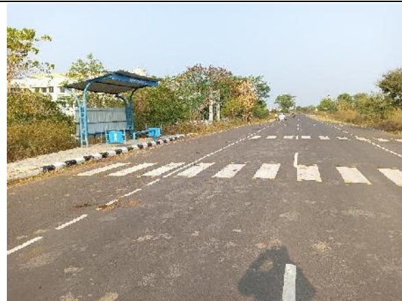
Bus Bay with Bus shelter @ Km 30.760-SH-296
