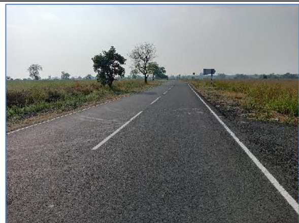
A view of Project Road Km: 29.600 -SH-296
