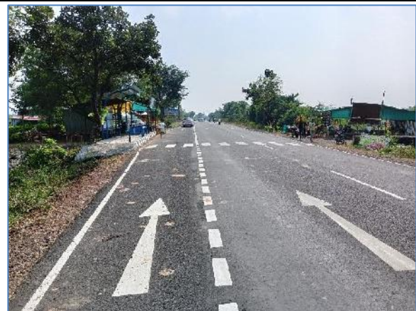
A view of Project Road Km: 23.400 -SH-297
