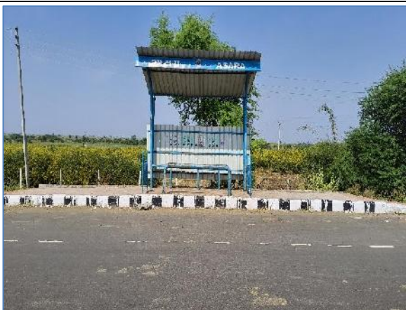
Bus Bay with Bus shelter @ Km 65.605-RHS
