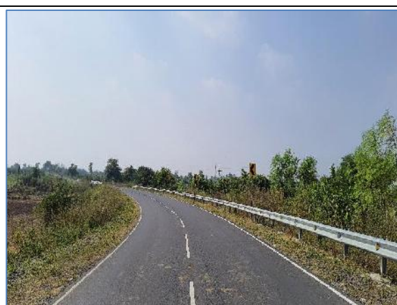
A view of Project Road at Km: 50.000_SH - 294
