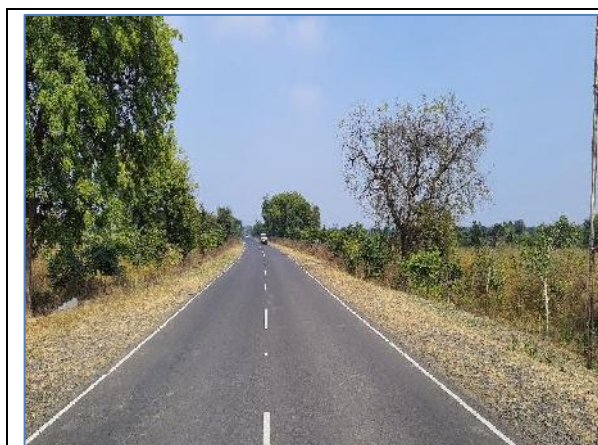
A view of Project Road at Km: 43.000_SH - 294
