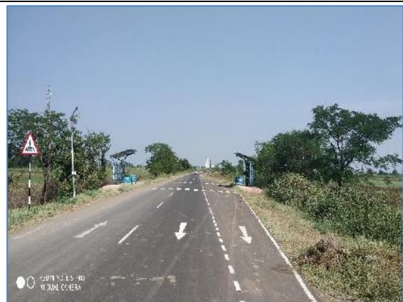
Bus bay with Bus shelter @ Km 71.650-BHS
