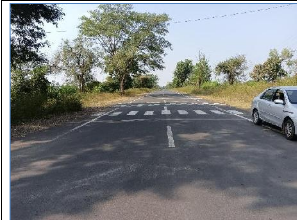
A view of Project Road Km: 1.675 Chandur Bypass
