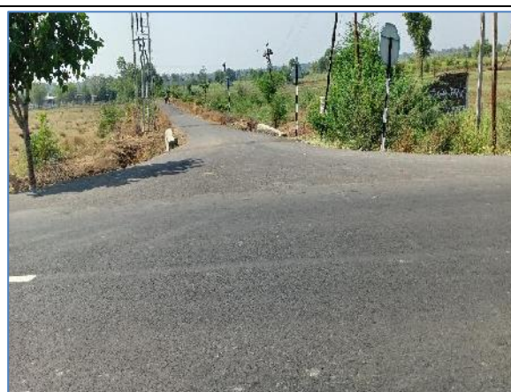
Minor Junction at km km 4+000 - RHS
