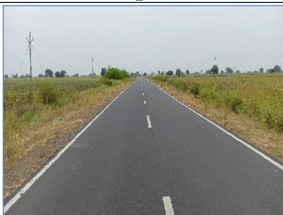
A view of the Project Road with 7.0m wide With at Km: 17.000_SH-280
