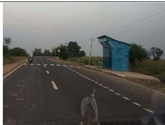
Bus Bay with Bus shelter @ Km 217.250-RHS
