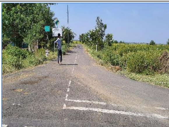
Minor Junction at km 69.145-LHS
