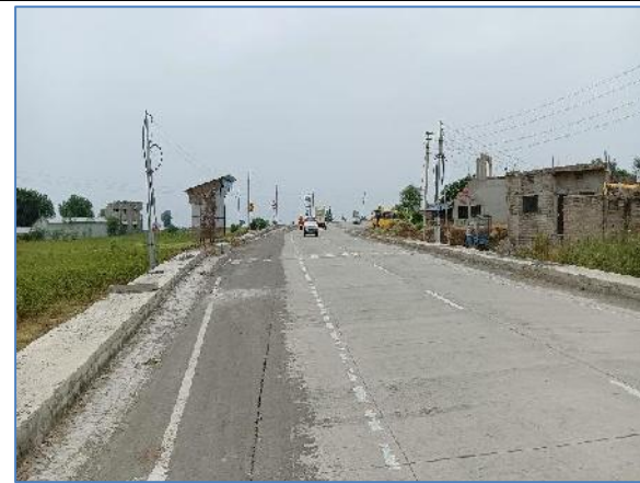
Bus Bay with Bus shelter @ Km 19.000-RHS_SH-280
