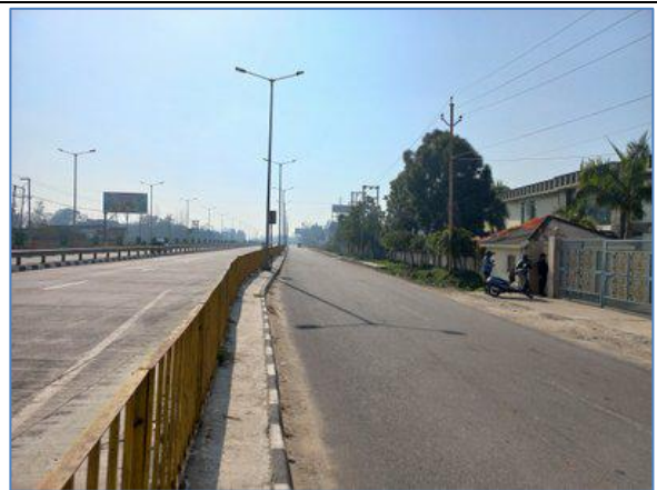
Service Road @ km 12.050 LHS - NH73
