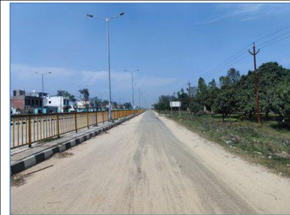
Service Road @ km 24.200 RHS - NH73
