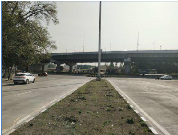
Major Junction @ km 0.000 LHS - NH-73
