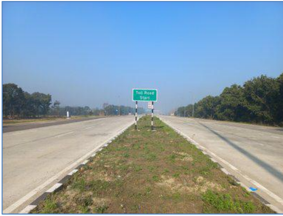
A view of the Project Road with Median 4m wide at km 0.000 - NH-73
