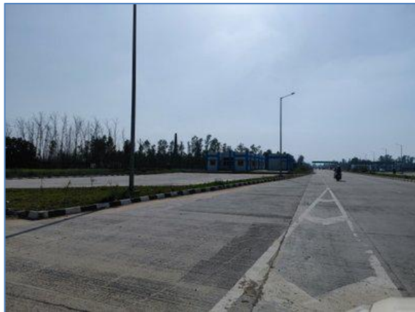
Truck Layby Cum Rest Area km 34.650 RHS - NH-73
