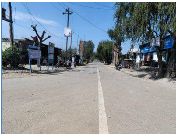
Minor Junction @ km 7.704 LHS - NH-72A
