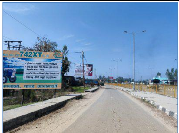
Service Road @ km 11.700 LHS - NH-72A
