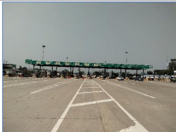
Toll Plaza @ 15+900 (Bhagwanpur Village)
