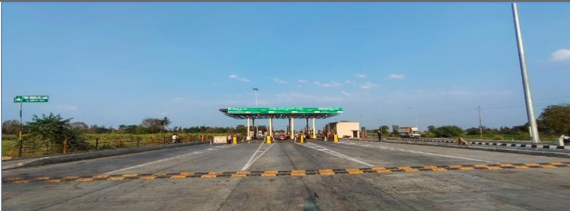
A view of the Toll Plaza near km 415+800-RHS
