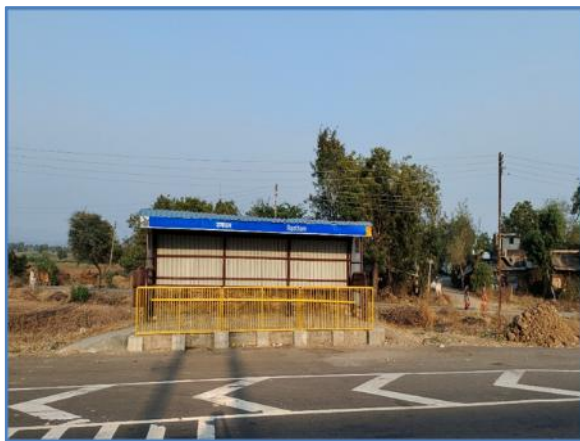
Bus Shelter near km 360.050 LHS
