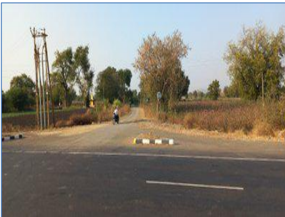
Minor Junction @ km 368.157 RHS
