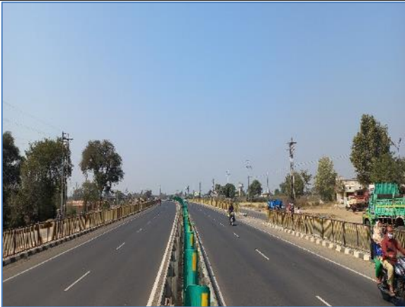
A view of the Project Road with Median 1.5m wide & MCB at Km 408.000
