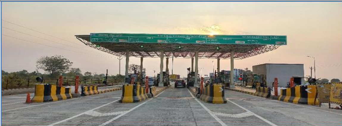
A view of the Toll Plaza near km 416+050-LHS
