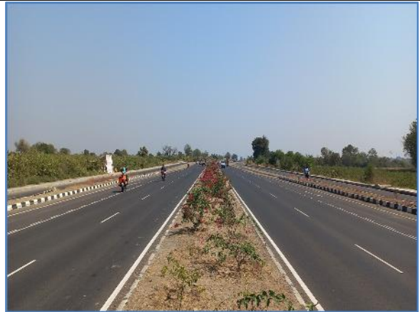
A view of the Project Road with median 4m wide at km 412.000
