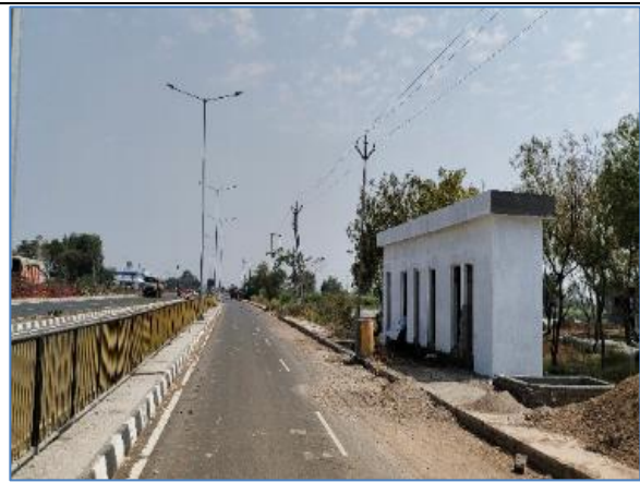
Truck Lay Bye Toilet Block @ Km 417.420 LHS
