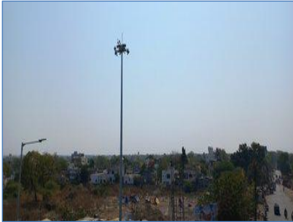
A view of High mast lighting @ km 404.010 LHS
