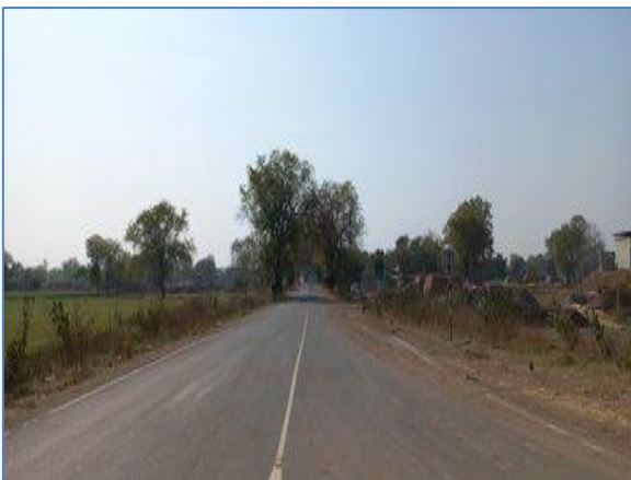
Major Junction @ km 387.240 LHS
