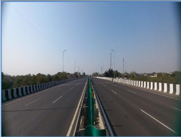
A view of the Project Road on Structure approach with Highway Lighting, CCB & MCB at Km 419.000
