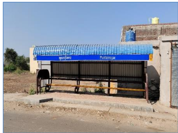
Bus Shelter near km 372.250 RHS
