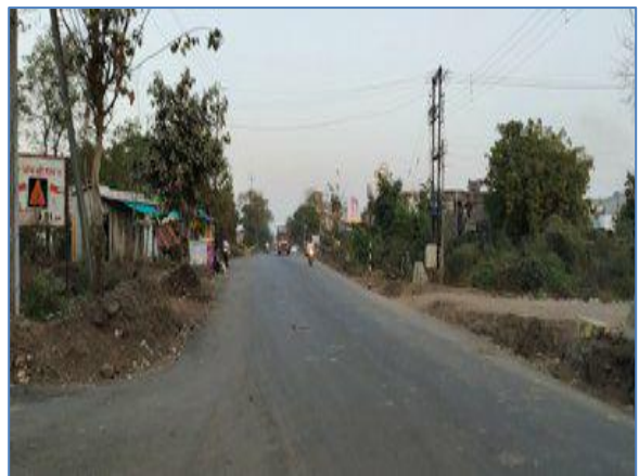
Minor Junction @ km 418.900 LHS
