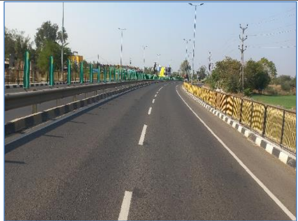
A view of the Project Road with PGR in SR Separator & MCB on Median at Km 420.000-RHS
