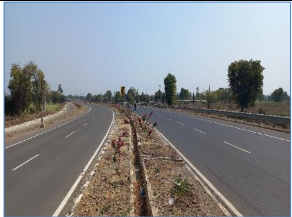
A view of the Project Road with Median Drain at Km 397.200
