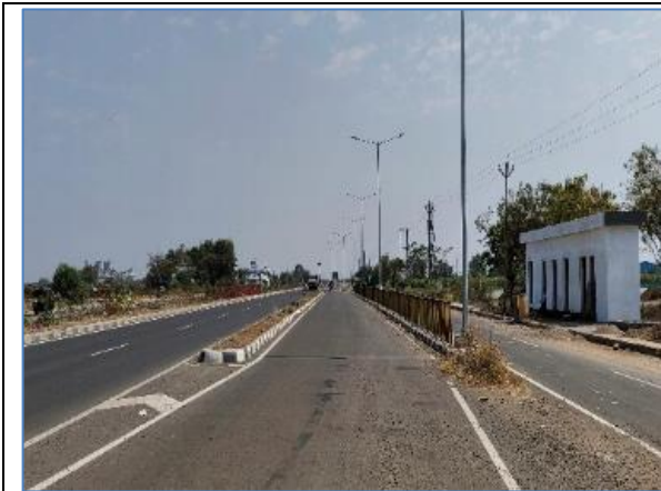
Truck Lay Bye @ Km 417.420 LHS
