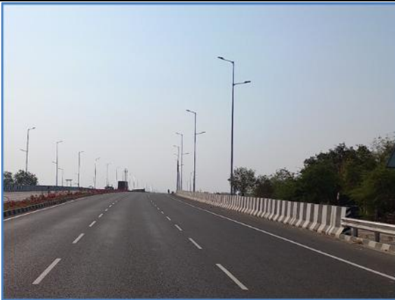
A view of the Project Road with 6-Lane Approach having Lighting, MCB & CCB at Km 381.000-RHS
