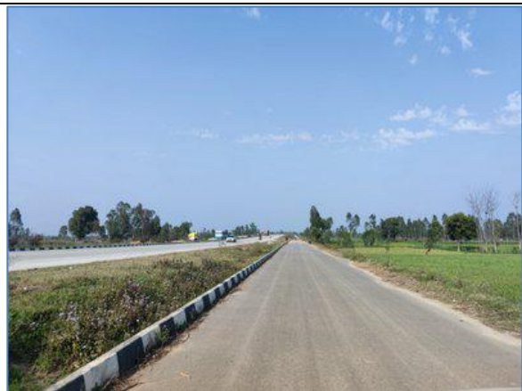
Service Road @ km 46.200 LHS - NH73
