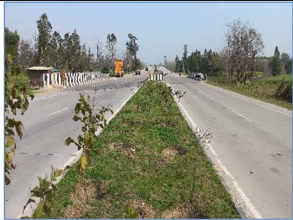
A view of the Project Road with Median 4m at Km 70.000 - NH-73
