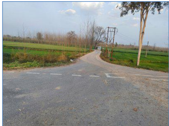
Minor Junction @ km 80.325 RHS - NH-73
