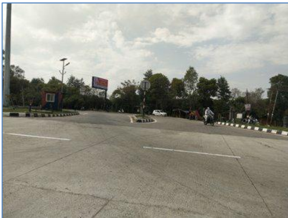
Major Junction @ km 36.288 RHS - NH-73
