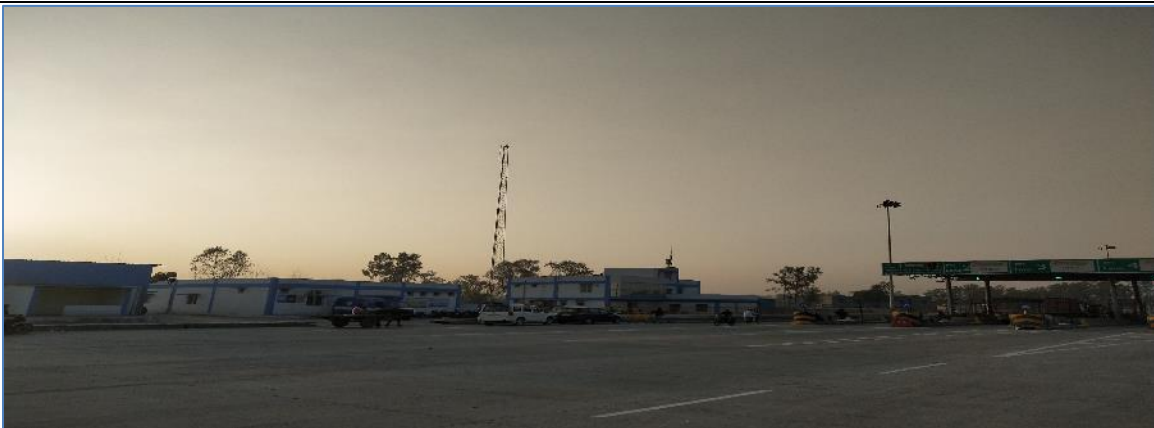
Admin Building at km.81.000
