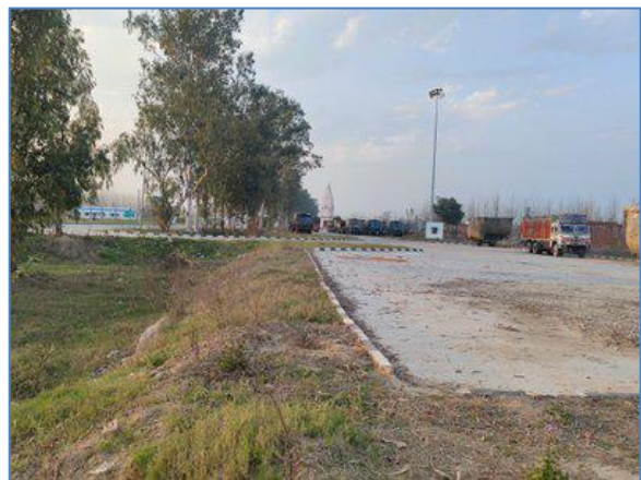
Truck lay bye cum rest area @ Km 80.000 RHS @ NH-73
