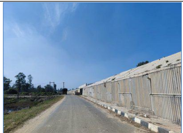
Service Road @ km 65.400 LHS - NH-73
