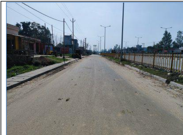
Service Road @ km 35.400 LHS - NH73
