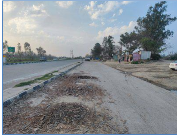
Truck lay bye near km 85.050 RHS - NH-73
