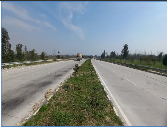
A view of the Project Road with Median 4m at Km 65.000 - NH-73
