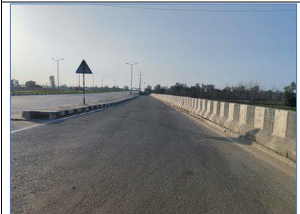
Service Road @ km 58.320 RHS - NH-73
