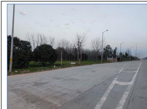
Bus Bay with Shelter near km 57.570 RHS - NH-72A
