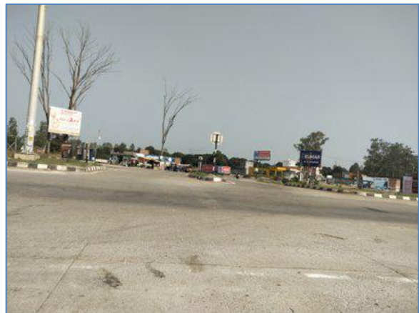
Major Junction @ km 79.682 RHS - NH-73
