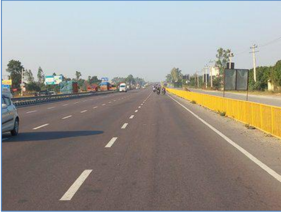
A view of the Project Road with PGR in SR Separator at Km 76.000-RHS
