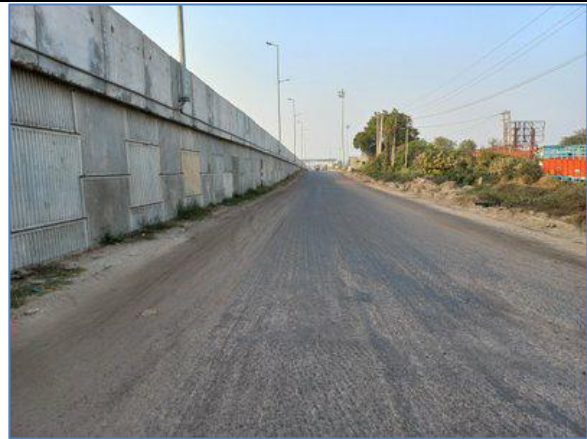
A view of Service Road with Double arm lighting near PUP km 53.400 RHS
