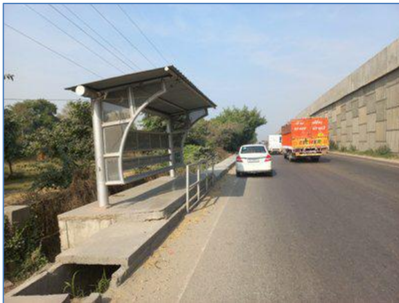
Bus Shelter near km 43.480 LHS
