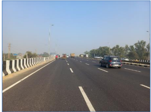
A view of the Project Road on Structure approach with Highway Lighting & CCB at Km 50.000-LHS
