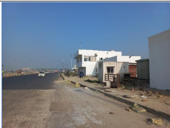
Admin Building at km.54.160 RHS
