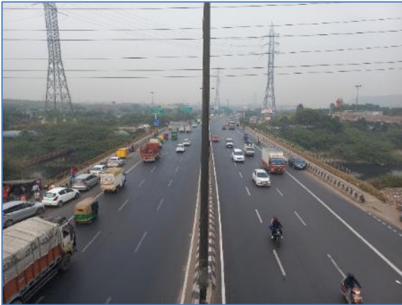
A view of the Project Road with median 1.2m wide at km 15.000
