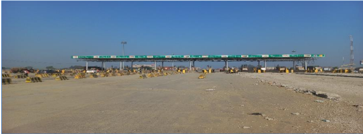
A view of the Toll Plaza near km 54.230 (Baghan)
