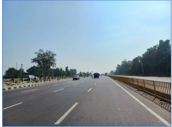
A view of the Project Road with MCB & PGR at Km 81.000-LHS
