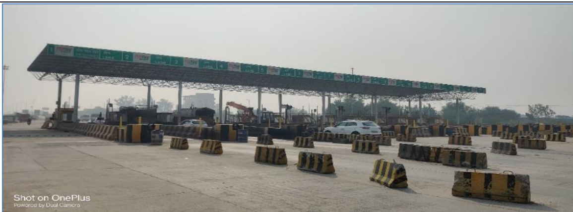
A view of the Toll Plaza near km 53.770 (Baghan)
