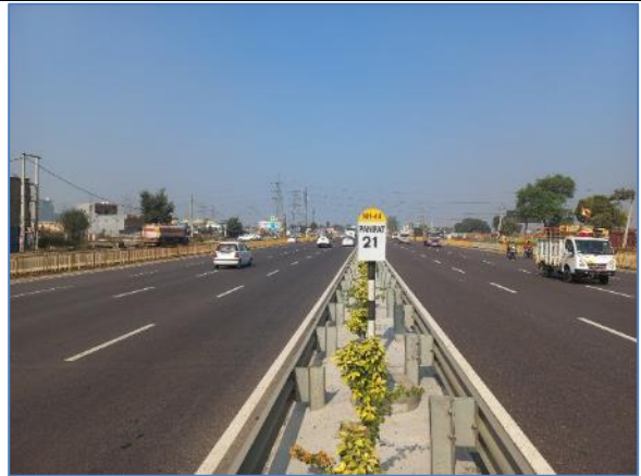
A view of the Project Road with Median 1.2m wide & MCB at Km 71.000-BHS
