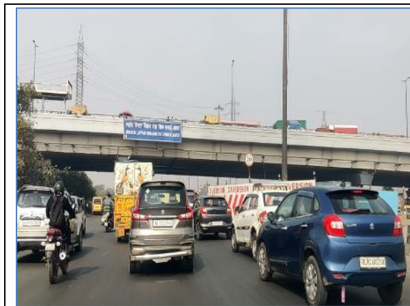
Start Point at km.15.000
