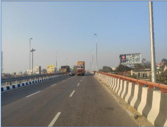
A view of the Project Road with 6-Lane Approach having Lighting, MCB & CCB at Km 62.000-RHS
