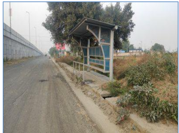
Bus Shelter near km 66.900 RHS
