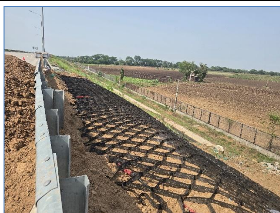
Repair works of Embankment at km 318.440 RHS
