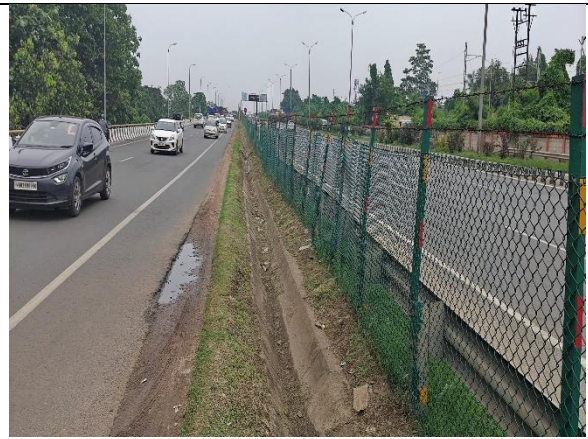
Drain at Km 655+300 LHS
