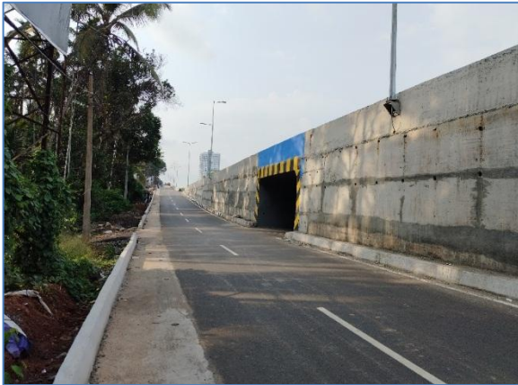
RCC closed drain at Km 247+200 RHS
