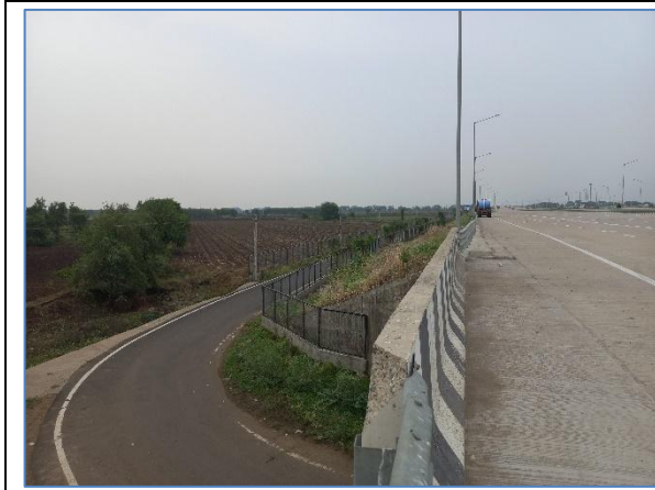
Connecting Road at km 317.500 LHS
