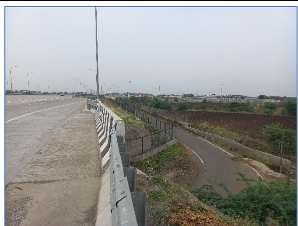
Connecting Road at km 318.980 RHS
