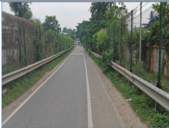
View of Ramp-E
