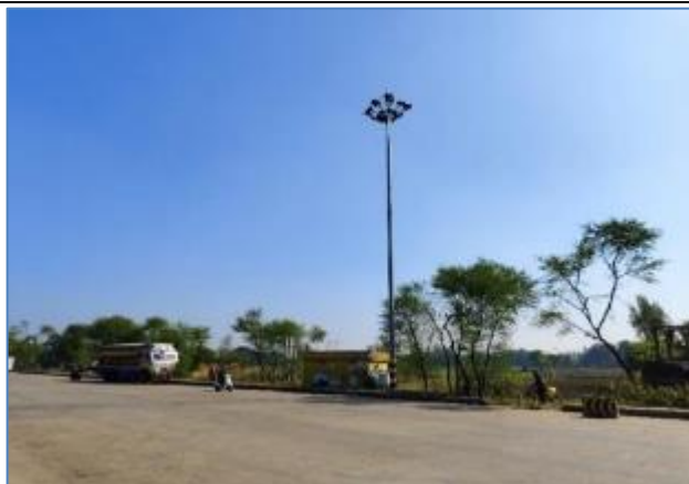
High-mast @ Km 216.500 LHS TP-1
