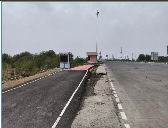
Static Weigh Bridge @ km 27.700
