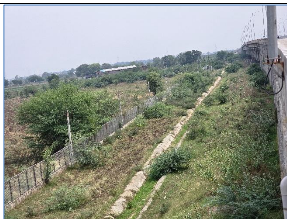
Trapezoidal Drain at km 292.600 LHS
