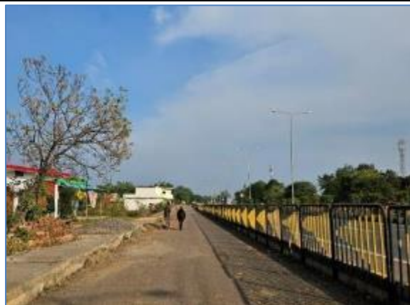
5.5m Wide service road @ Km 182.500 LHS
