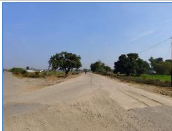
Minor Junction @ Km 222.490 LHS
