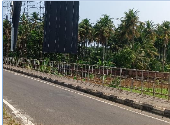
RCC drain cum Footpath at km. 258+793 RHS
