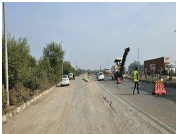
Truck lay-bye @ km 221.700 RHS
