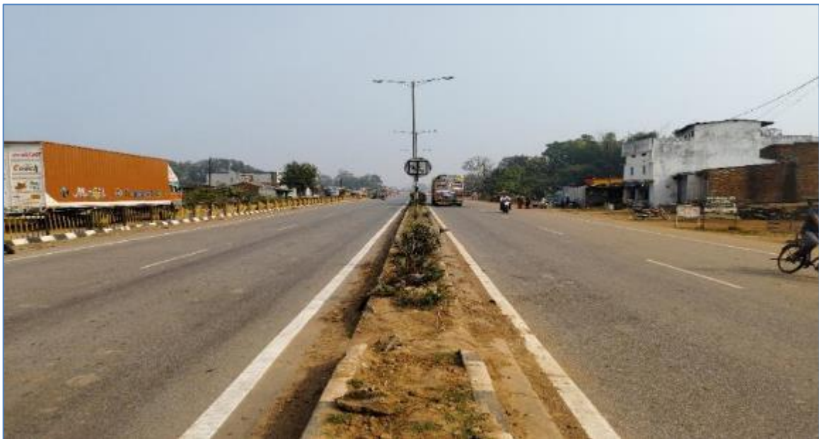
A view of the Project Corridor with 9.5m wide carriageway on both sides of 1m wide Median at Km 158.000
