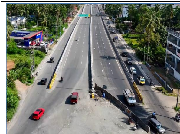
Start Point of the Project at Km. 230.400
