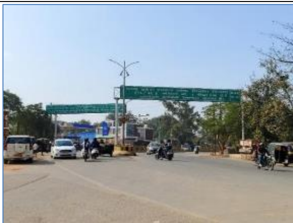
Major Junction @ Km 229.850 LHS
