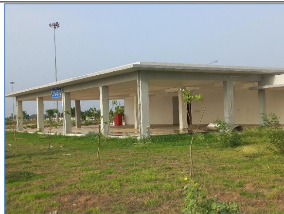
Dhaba at km 306.500 LHS Rest Area
