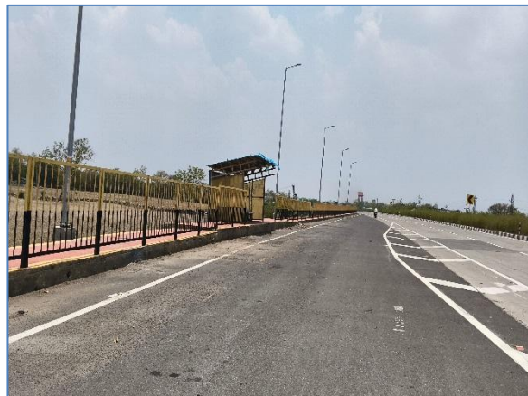
Bus Bay with Bus shelter @ 22.000 LHS
