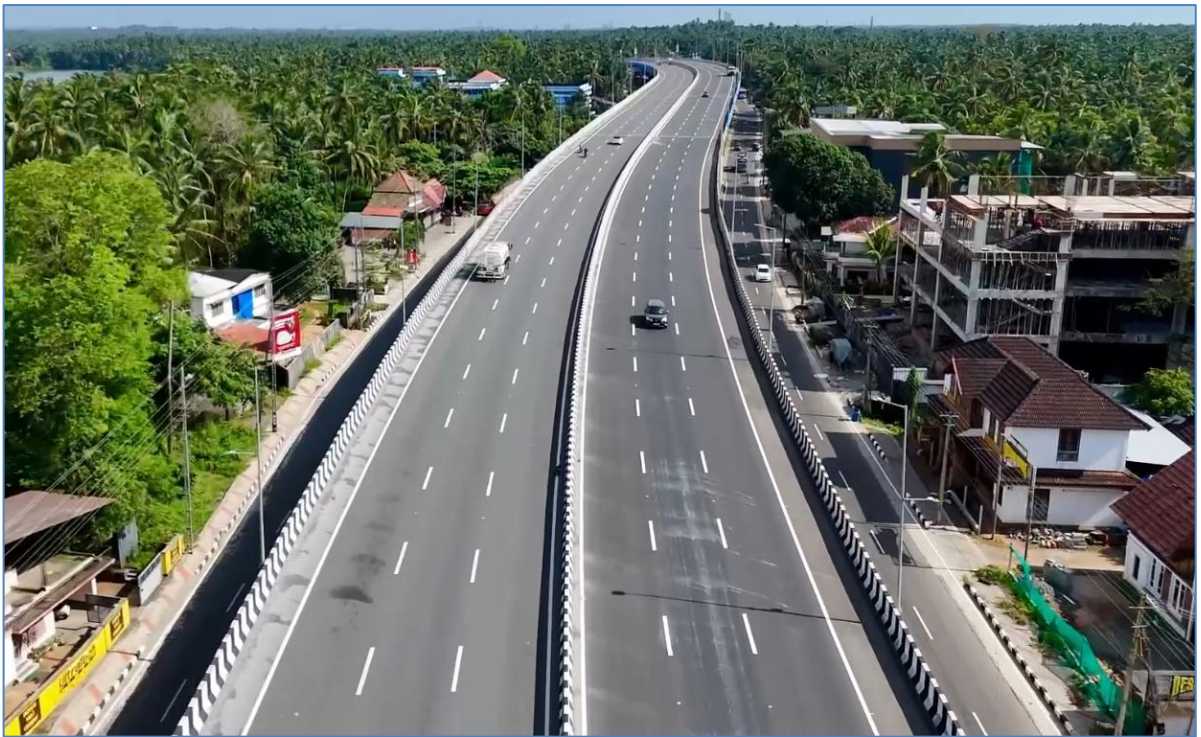
View of the Project corridor at Km. 231+000 with a 6-lane configuration in the main carriageway (MCW) with Segmental Arm Lights on Shoulders and provided with CCB on Median.
