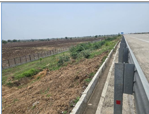
Lined Drain at km 302.900 LHS
