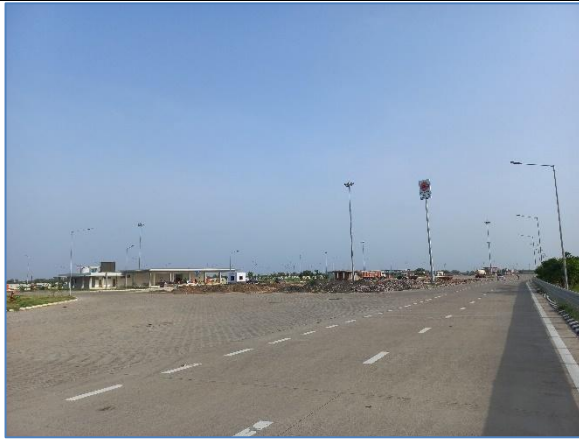
Rest Area at km 306.500 LHS
