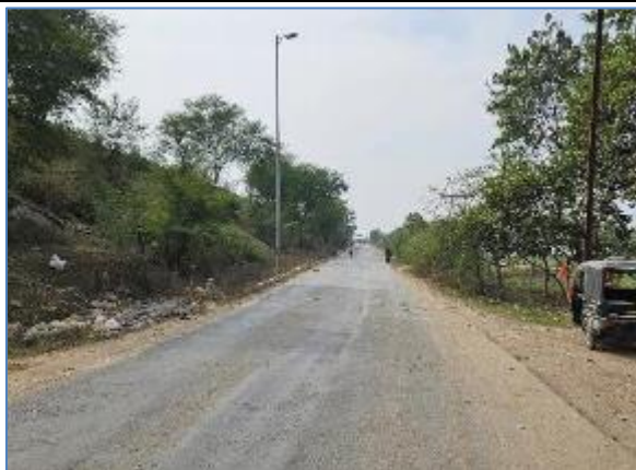
7m wide Service Road at Km 205.700 RHS
