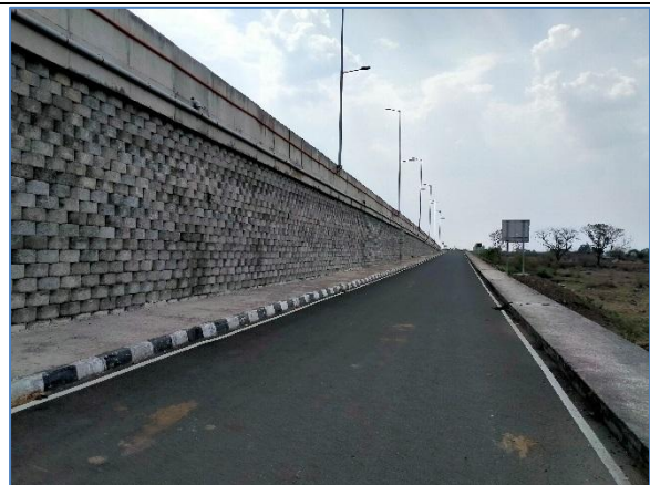
Service road at km 45.800 RHS
