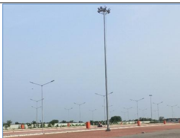
High mast at km 306.530 LHS
