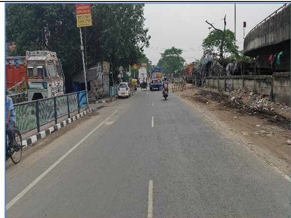
View of PWD-Down road
