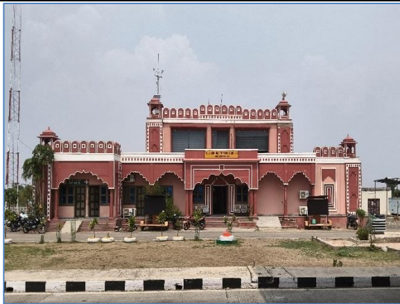
Toll Admin Building @ km 27.700
