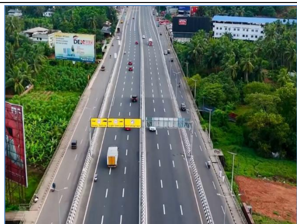
End Point of the Project at Km. 258.800
