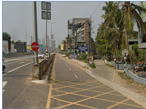
Minor Junction @ km 251.160 LHS
