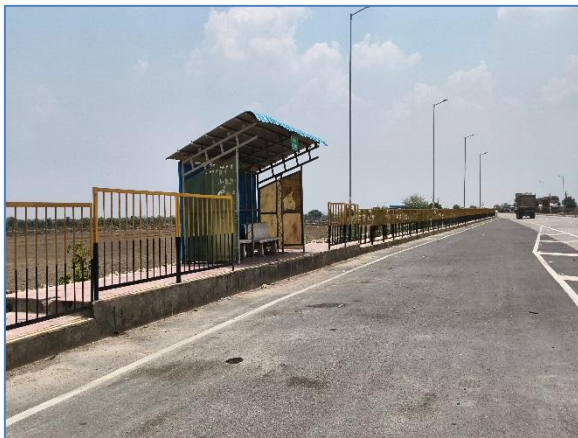
Bus Bay with Bus shelter @ Km 13.550 RHS
