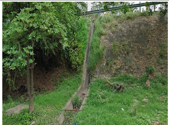
High Embk. with chutes km 653+600 RHS
