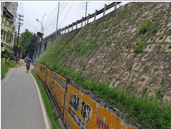
Partial RCC wall Km 655+160 LHS
