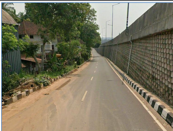
5.5m wide Slip Road @ Km 243.500 LHS
