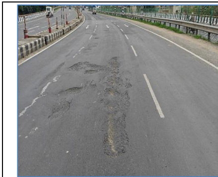
Delamination @ 656.000 LHS
