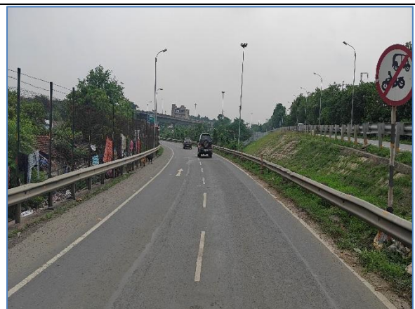
High Mast Lighting at km 658.000 Ramp-B
