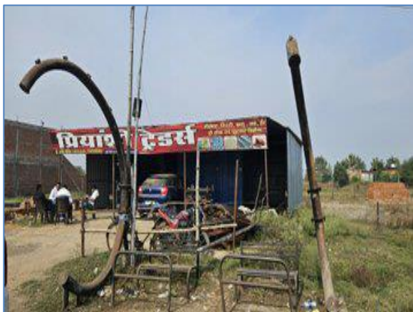
damaged Bus shelter @ km 170.900 RHS
