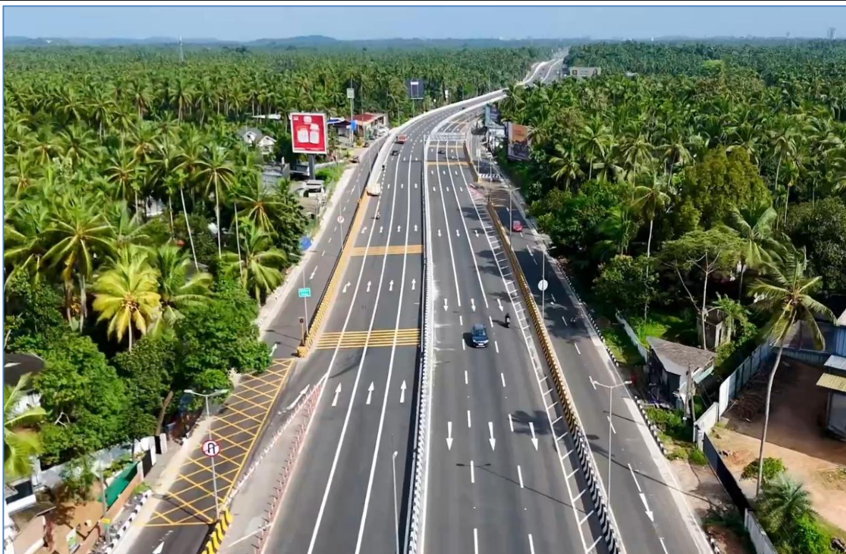
View of the Project corridor at Km. 237+000 with Entry to MCW from Service Road
