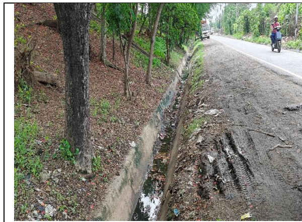
Drain at Km 653+500 RHS
