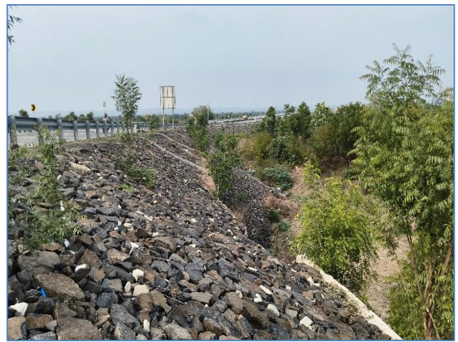
Stone Pitching at km-56+900 RHS
