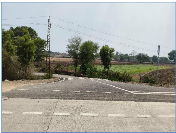
Minor Junction at km 32.550 BHS
