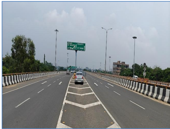
A view of stretch at km 657.910
