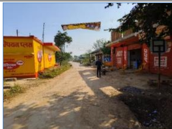
Minor Junction @ Km 226.400 LHS
