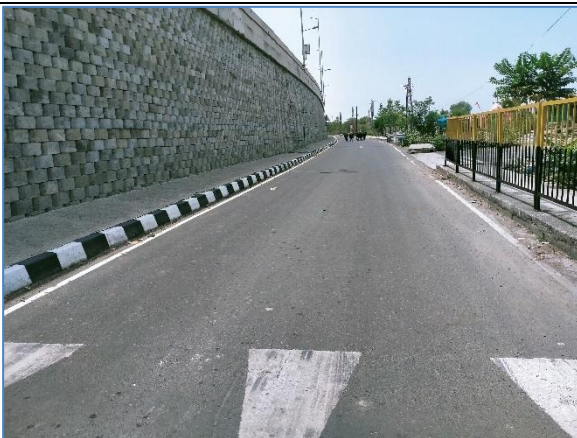
Service road at km 24.600 LHS
