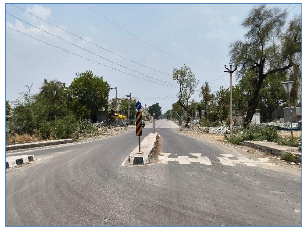
Major Junction at km 27.000 BHS
