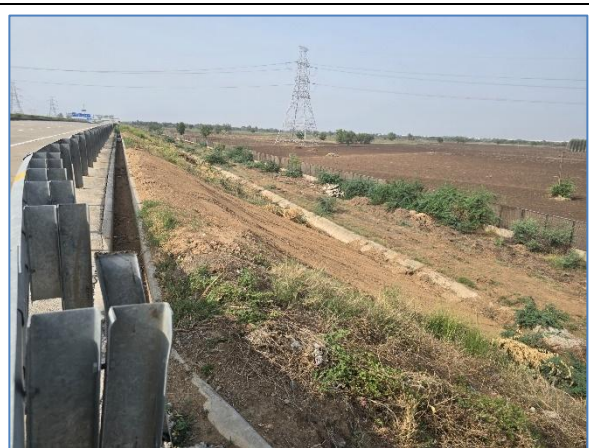
RE Blocks at km 299.350 LHS
