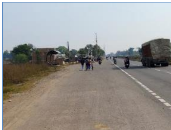
Bus-bay with shelter @ km 218.920 RHS
