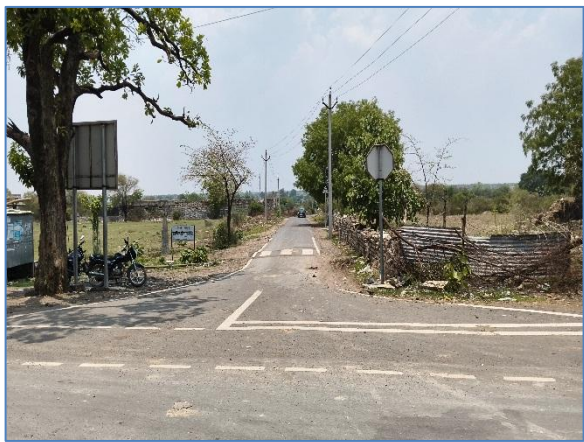
Minor Junction at km 19.900 BHS
