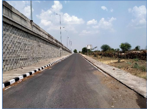
Service road at km 38.500 RHS
