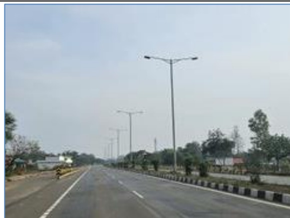
Double Arm Lighting @ Km 182.600 Median
