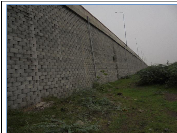
RE Blocks at km 299.350 LHS
