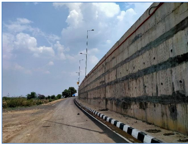
RCC Wall at km-32+600 RHS
