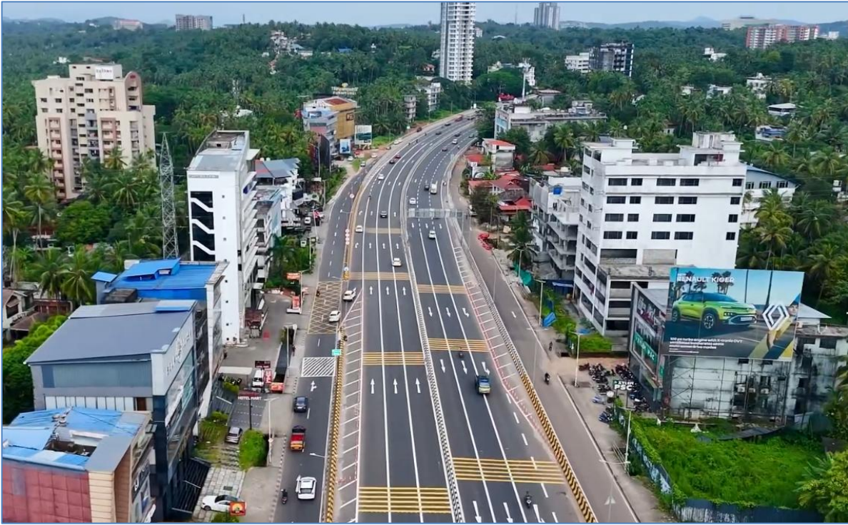
A View of Project Corridor with Slip Roads @ km 246+100 in Built-up Area
