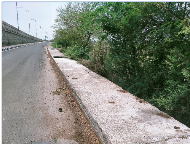
RCC Cover Drain at Km 12+550 LHS
